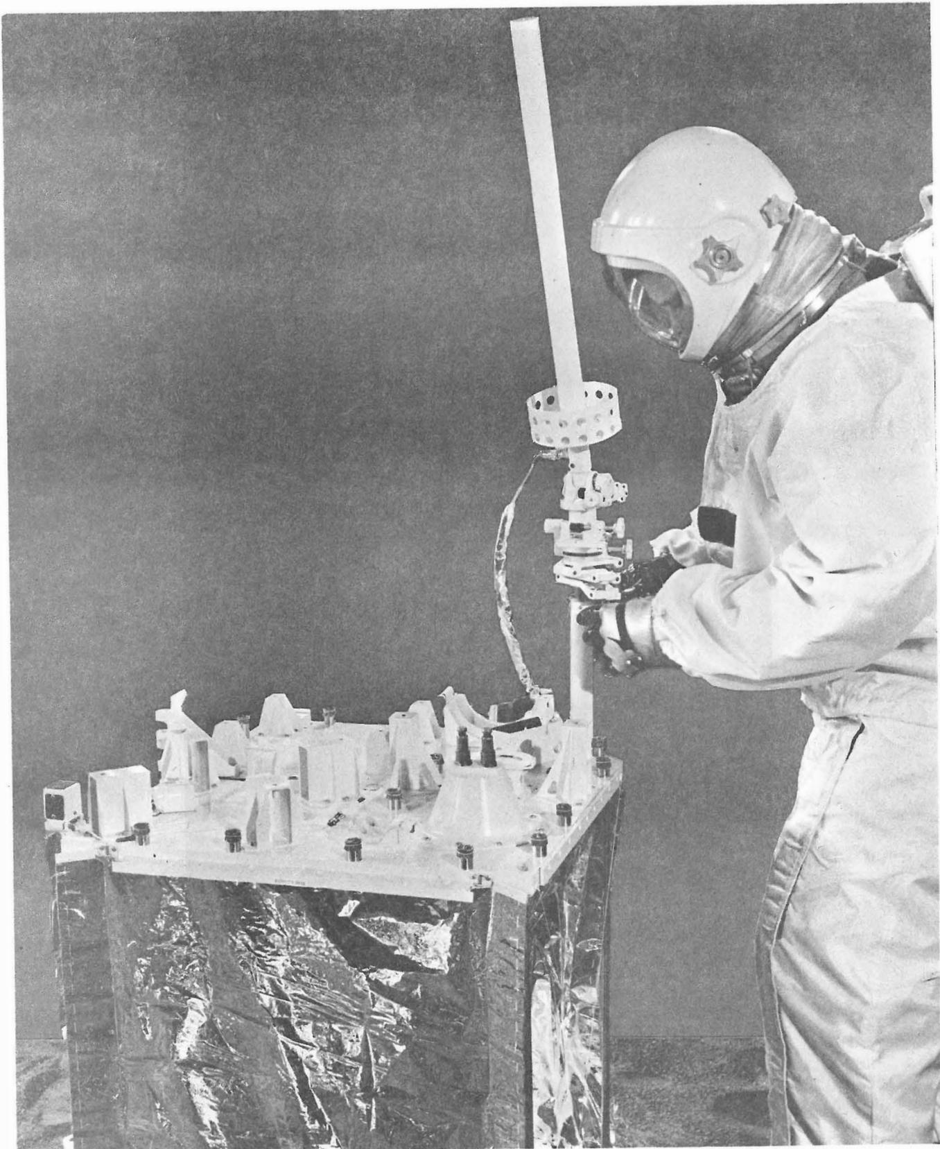
Figure 4-9. Antenna Aiming Mechanism Alignment
