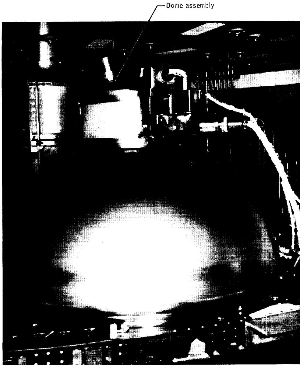
Figure D3-20.- Oxygen shelf showing location of tank dome assemblies.
