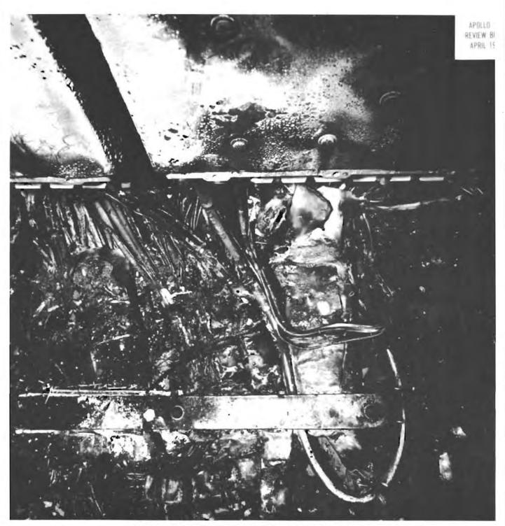
VIEW OF AFT BULKHEAD WIRING BELOW INVERTERS
