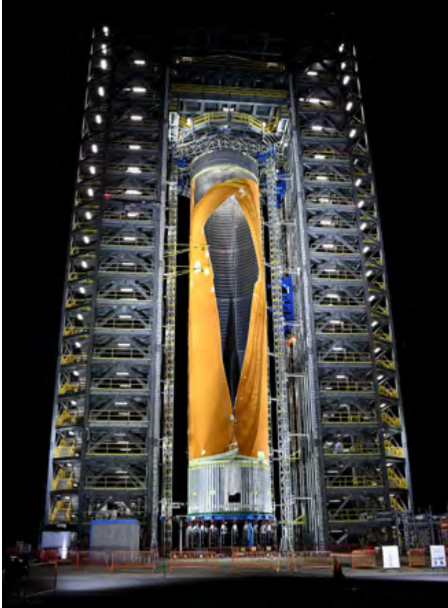
▲ The SLS liquid hydrogen tank is pushed to its limits on Dec. 5, 2020, to see how much force it would take to cause the tank's structure to fail. This image shows the resultant buckling of the structure when the tank failed after exposure to more than 260% of expected flight loads over 5 hours. Image credit: NASA
