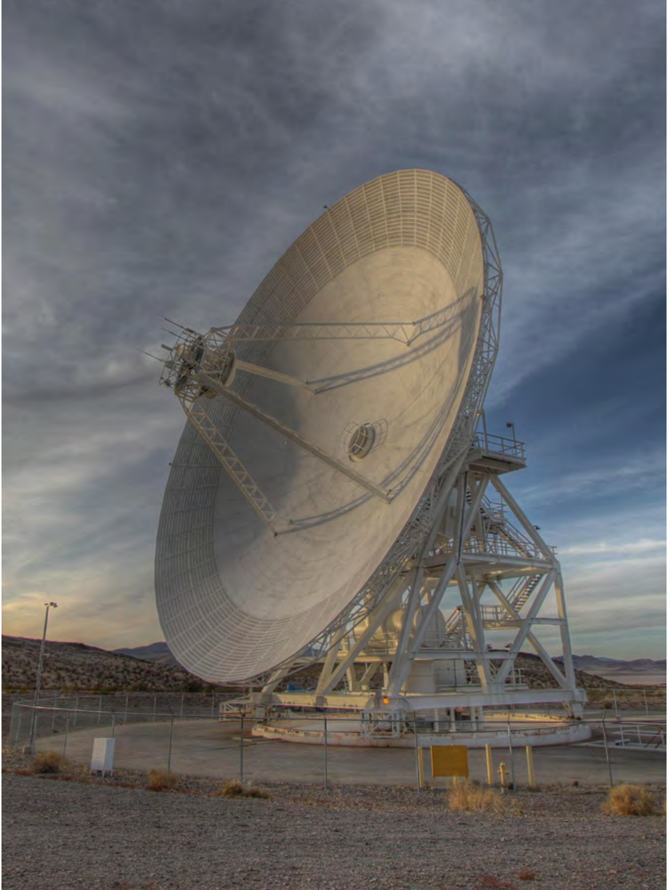
▲ A Goldstone 111.5-foot (34-meter) Beam Waveguide antenna tracks a spacecraft as it comes into view. The Goldstone Deep Space Communications Complex is located in the Mojave Desert in California. Image credit: NASA
