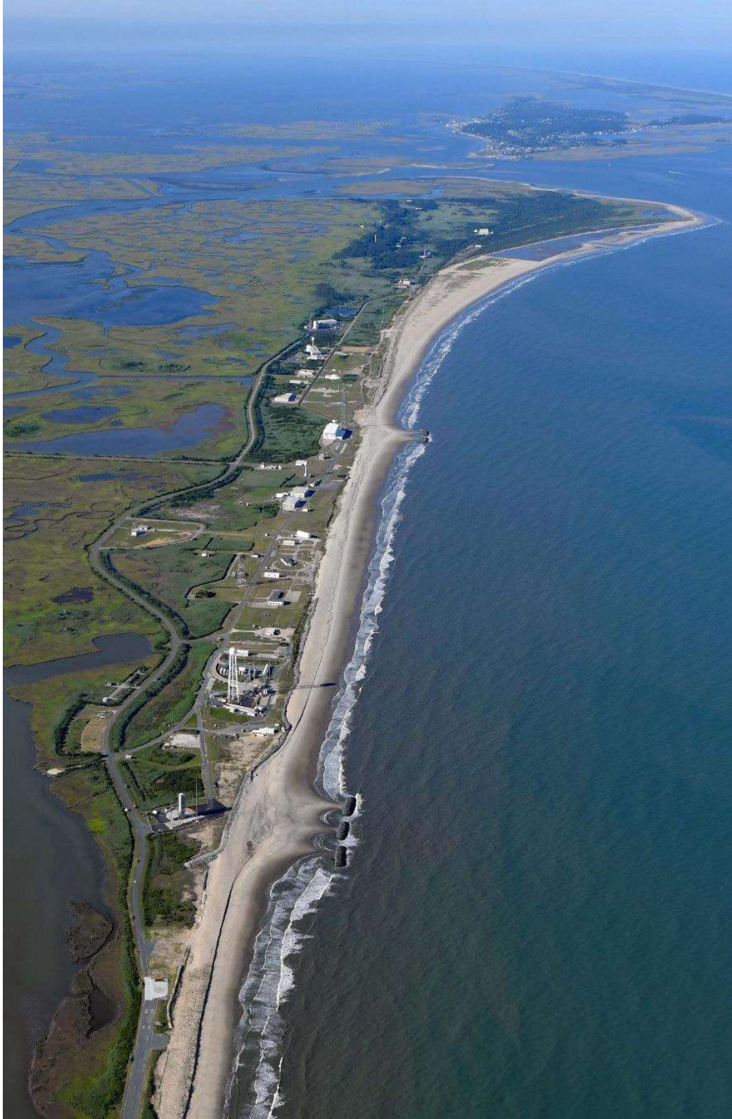
Figure 2 Shoreline Infrastructure Protection Area in 2021 After Breakwater Construction and Renourishment (Photo courtesy of Patrick J. Hendrickson)
