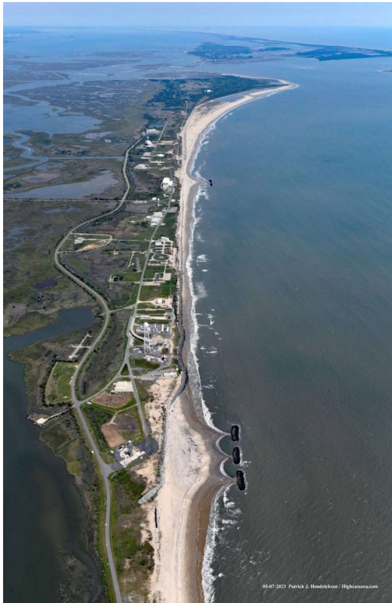
Figure 1 Wallops Island Infrastructure Protection Area in 2023
