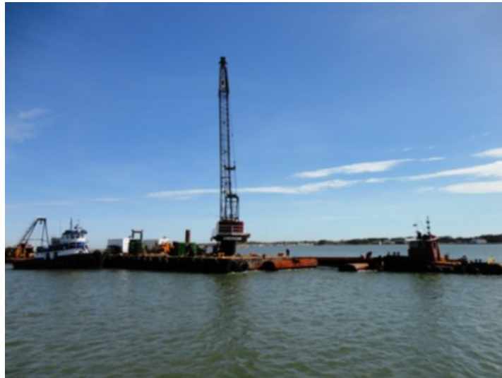
Figure 2-2 Beach Fill Offshore Equipment
