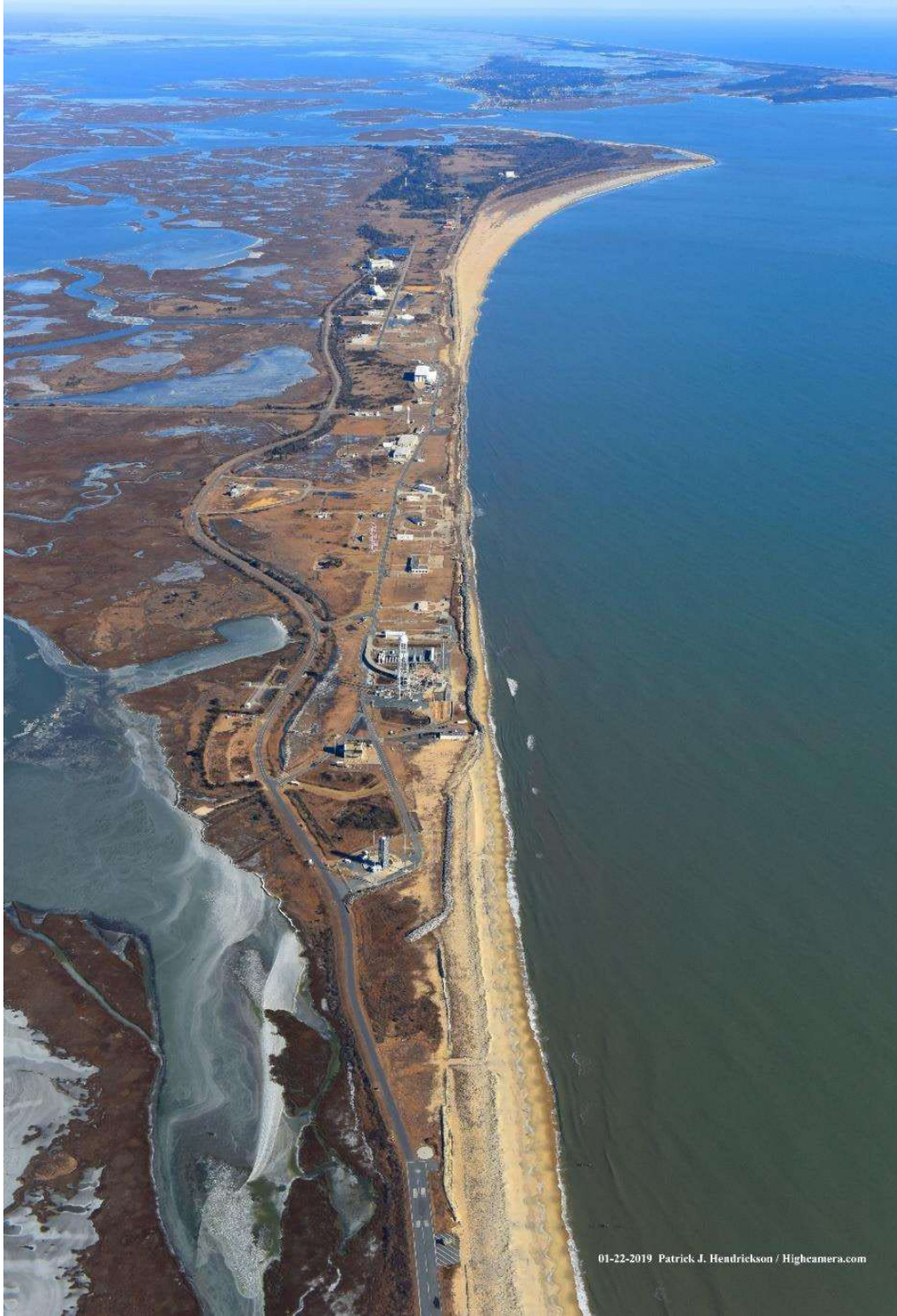
Figure 1 Shoreline Infrastructure Protection Area in 2019 Before Breakwater Construction and Renourishment (Photo courtesy of Patrick J. Hendrickson)
