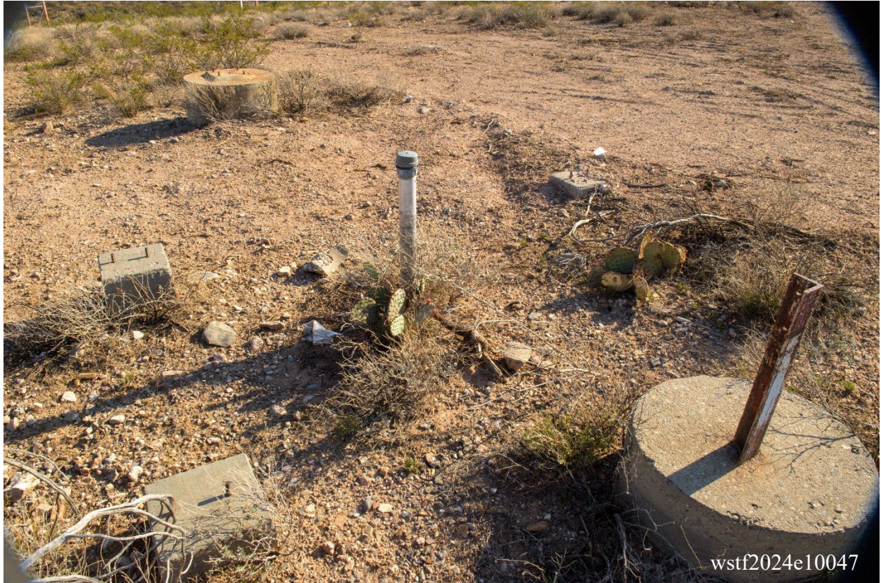
Figure 6 – Concrete pads with anchor bolts are the base mount of the burner and stack, and the white pipe is the electrical conduit. The metal stands on concrete were the piping mounts.
