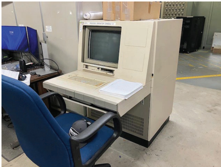
Figure 22. Peripheral control monitor for Chamber B to be removed and excessed.
