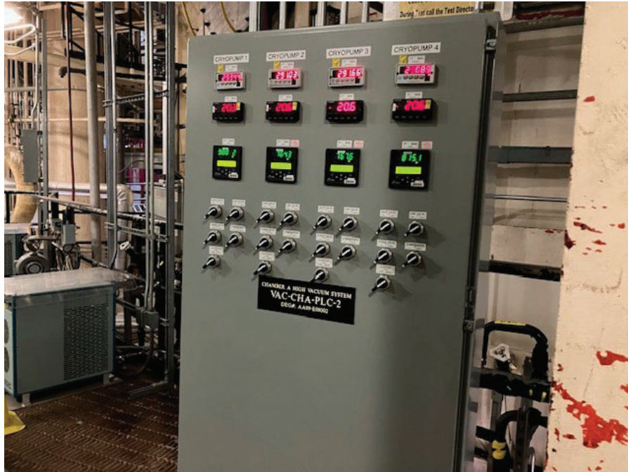
Figure 7. Cryopump controls previously installed next to Chamber A, for reference.
