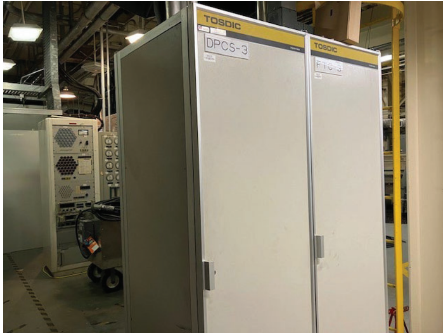
Figure 19. Additional peripheral control consoles for Chamber B to be removed and excessed.
