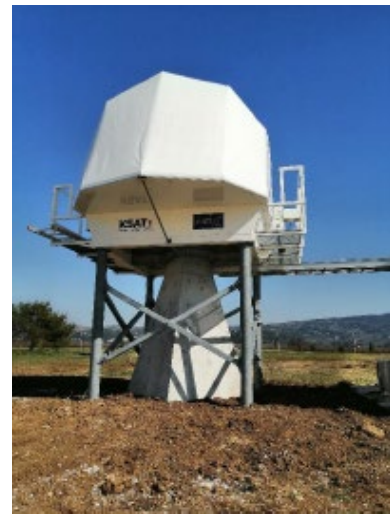
Figure 11.38: KSAT's low-complexity optical ground station in Nemea (2021).
