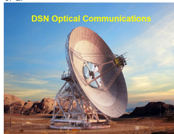
Figure 11.37: Artist overlay of built DSN RF antenna and planned 8m optical segments at its center. Credit: NASA.
