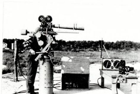
Modified Mk 51 Gun Director Used As Phototheodolite on Grebe Range
