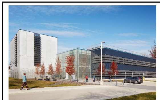
The Aerospace Communications Facility, recently completed at GRC, is comprised of approximately 25 laboratory spaces, including a large high-bay research space, along with rooftop and ground-based antenna fields. The new building with state-of-the-art capabilities supports development of specialized aerospace communication technologies for the agency.
