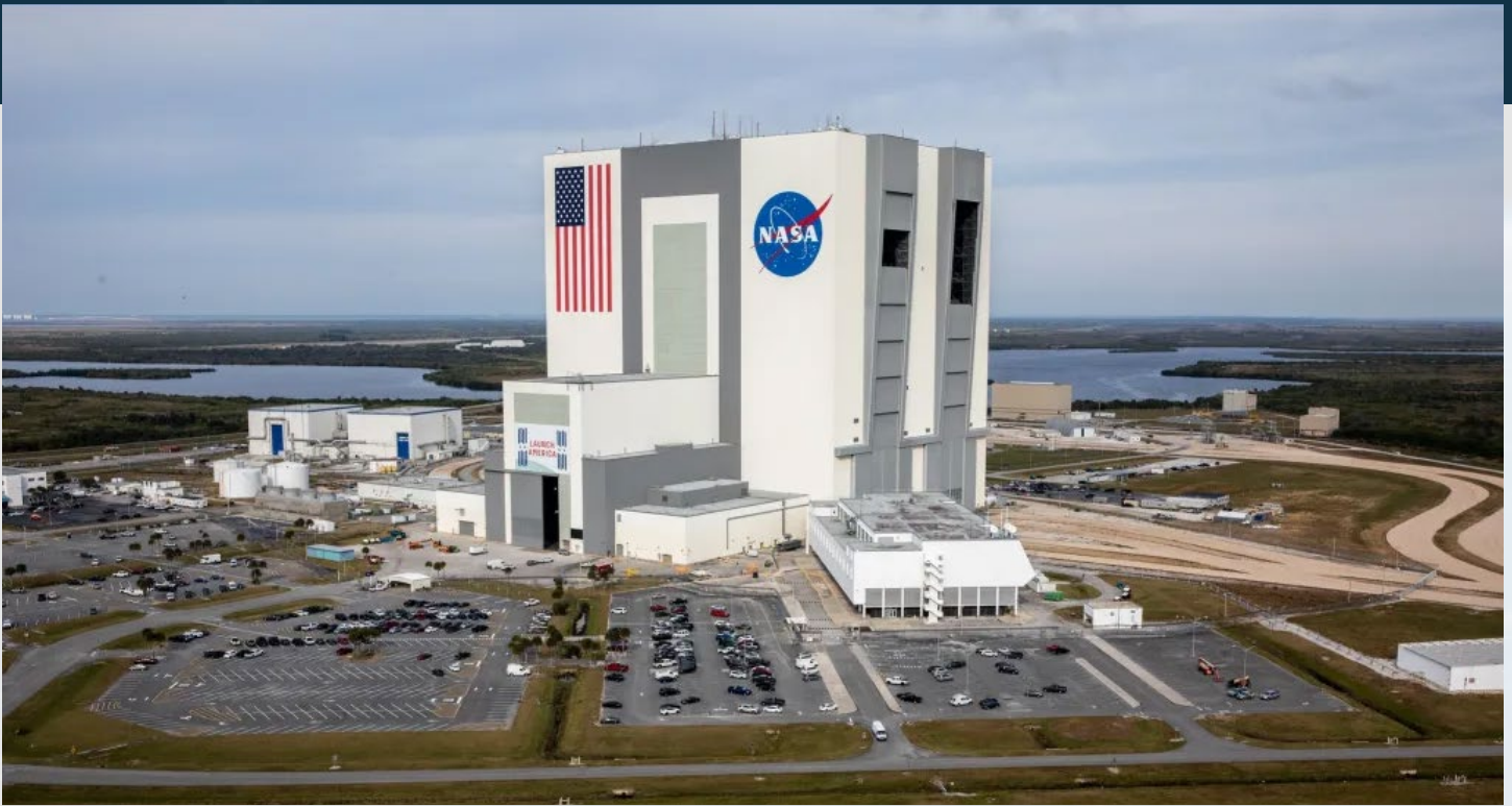
Photo of NASA's Kennedy Space Center Vehicle Assembly Building in Florida.
