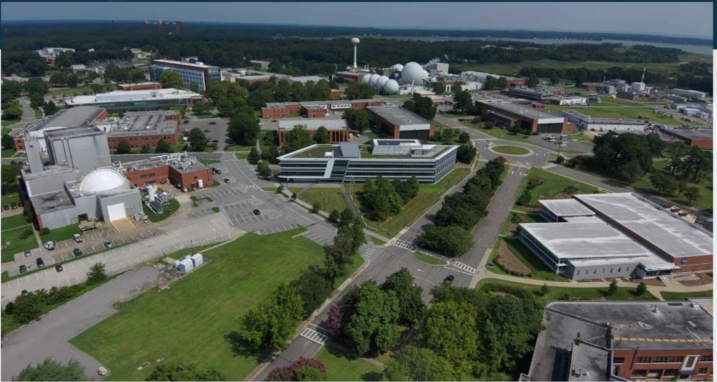
Aerial photo of NASA's Langley Research Center in Virginia.
