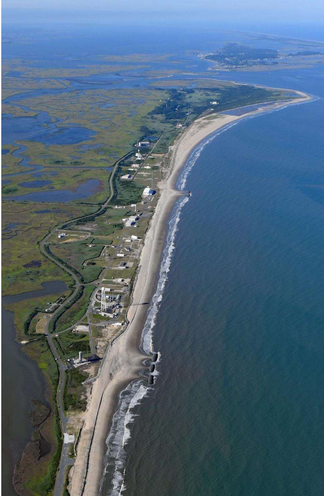
Figure 1.2-2 Shoreline Infrastructure Protection Area in 2021 After Breakwater Construction and Renourishment (Photo courtesy of Patick J. Hendrickson)
