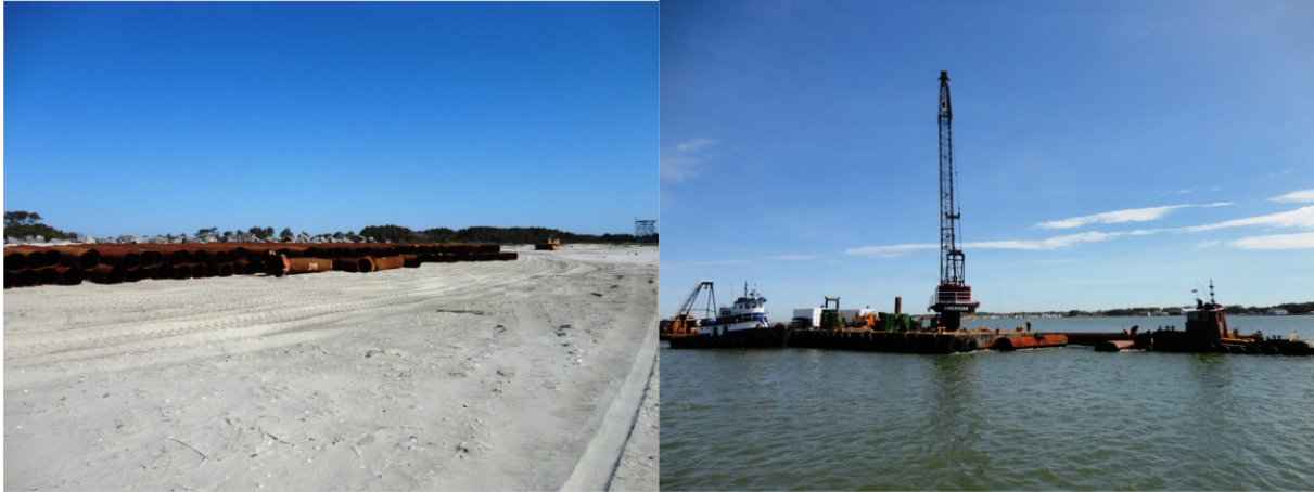
Figure 2.2-2 Beach Fill Mobilization/Onshore Staging (left) and Offshore Equipment (right)
