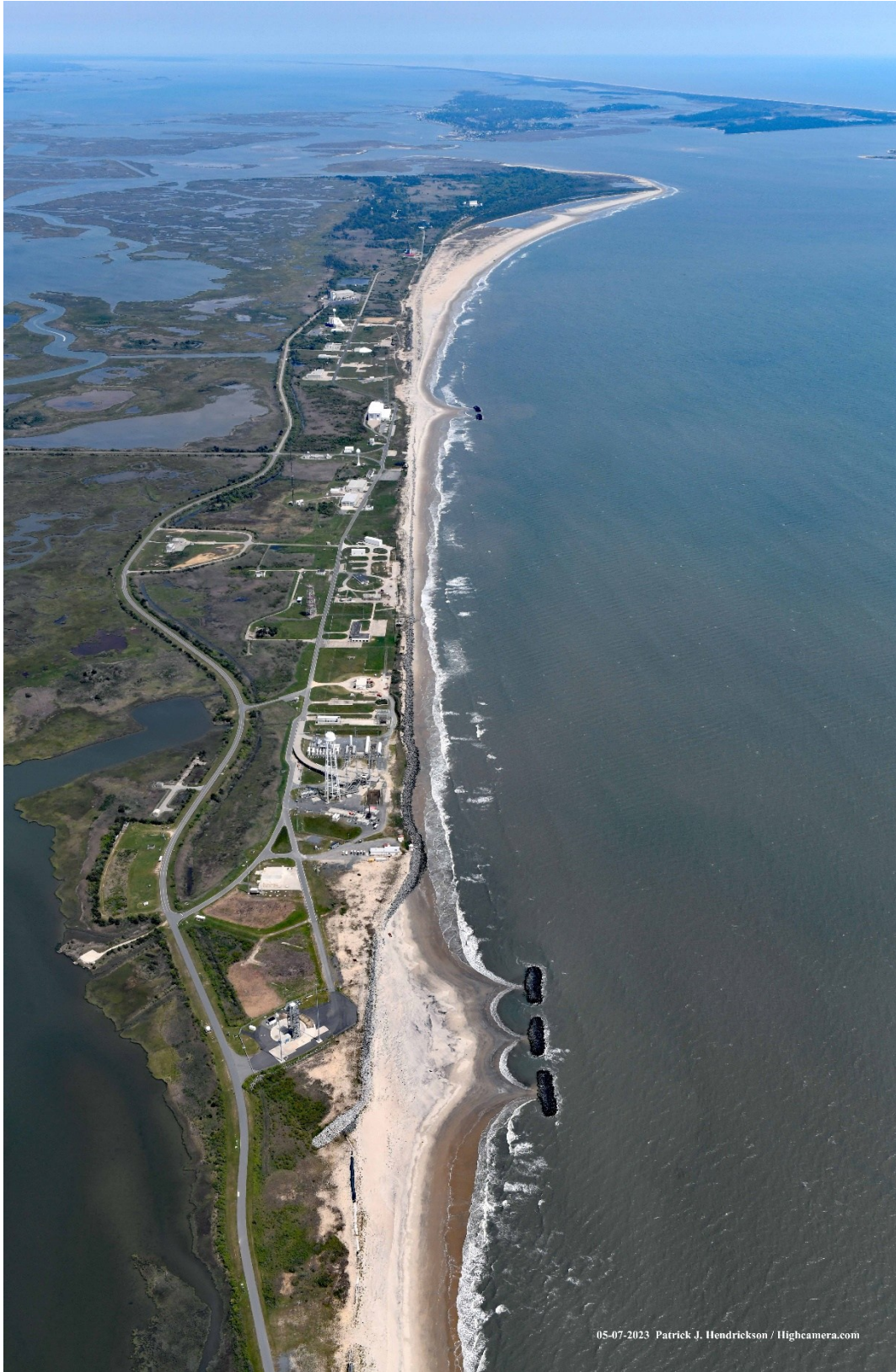
Figure 1.2-3 Shoreline Infrastructure Protection Area in 2023 (Photo courtesy of Patrick J. Hendrickson)
