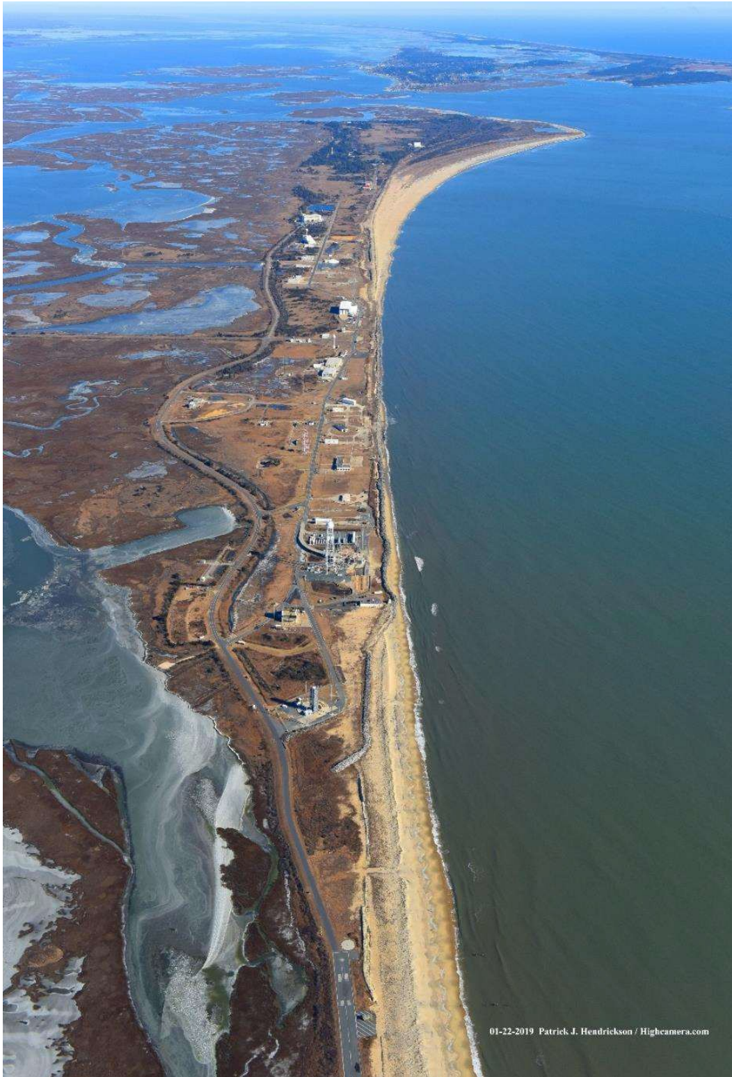
Figure 1.2-1 Shoreline Infrastructure Protection Area in 2019 Before Breakwater Construction and Renourishment (Photo courtesy of Patrick J. Hendrickson)
