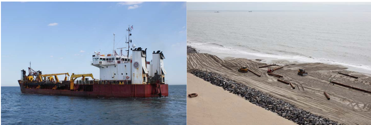
Figure 2.2-3 Dredging and Sand Placement Process with Trailing Suction Hopper (left) and Bulldozers Grading Discharged Sand (right)
