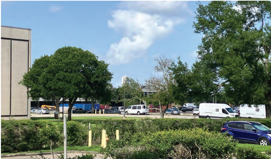
Looking northeast from B8 toward proposed B31 Renewal (visible; mostly obscured by B31X and mature trees)
