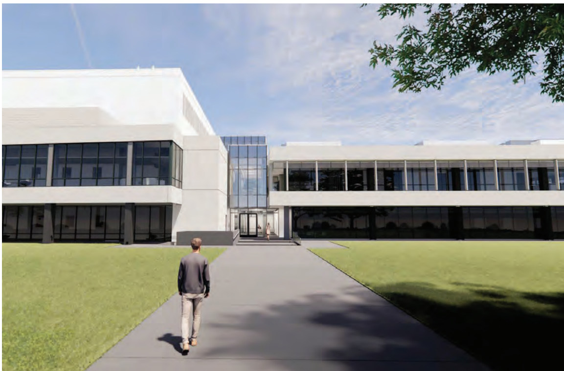
South Façade showing second and third floor Link with new West wing behind
