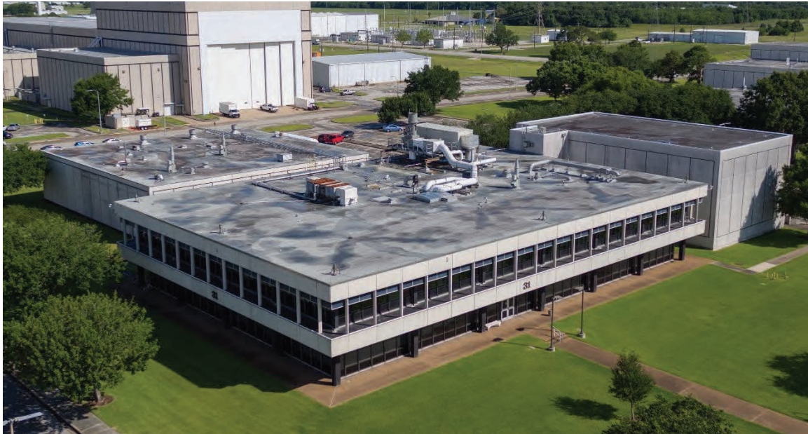
B31E (front) and B31N (right) with B31W behind (left) before B31X construction
