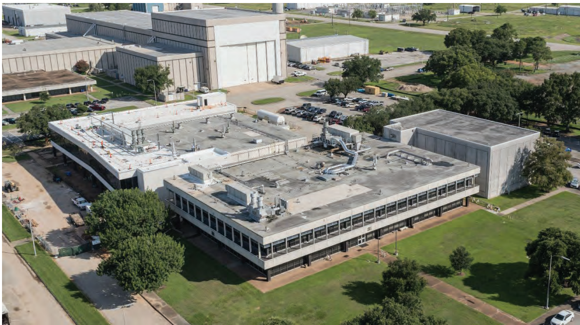
B31E (front) and B31N (right) with B31W and B31X, nearing construction completion, behind (left)
