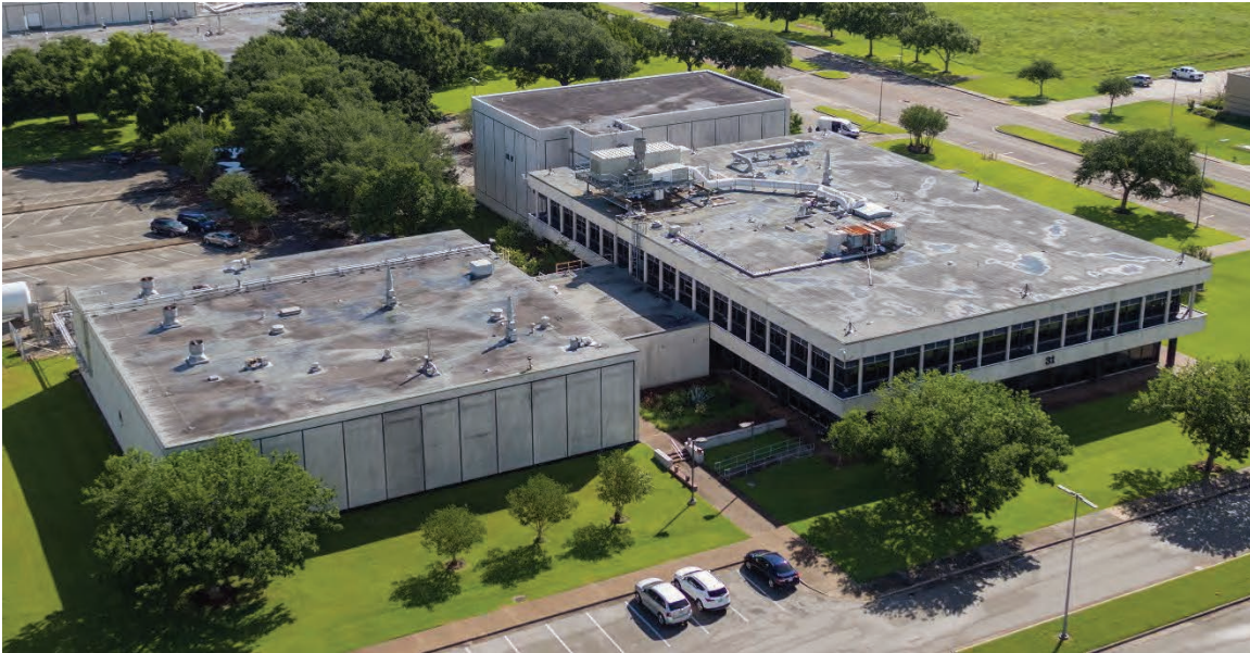
South façade of B31W (left) before B31X construction
