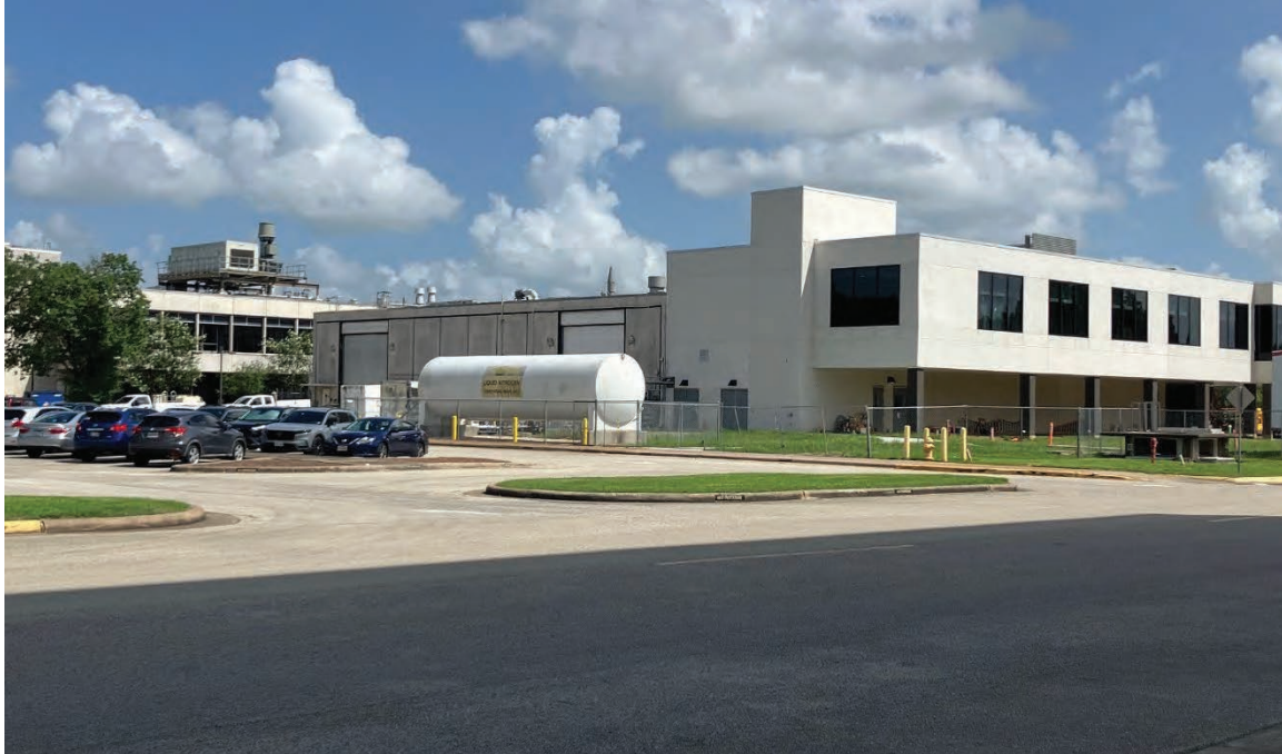
Looking east from B9 toward proposed B31 Renewal (visible; partially obscured by existing equipment and B31X)
