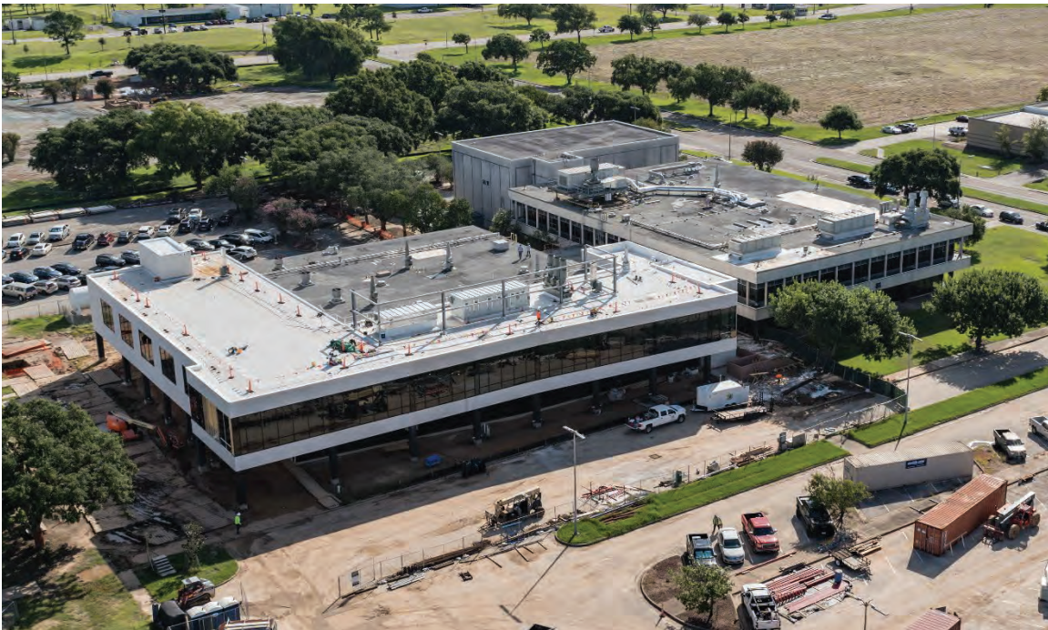
South façade of B31X (nearing construction completion) with B31W behind
