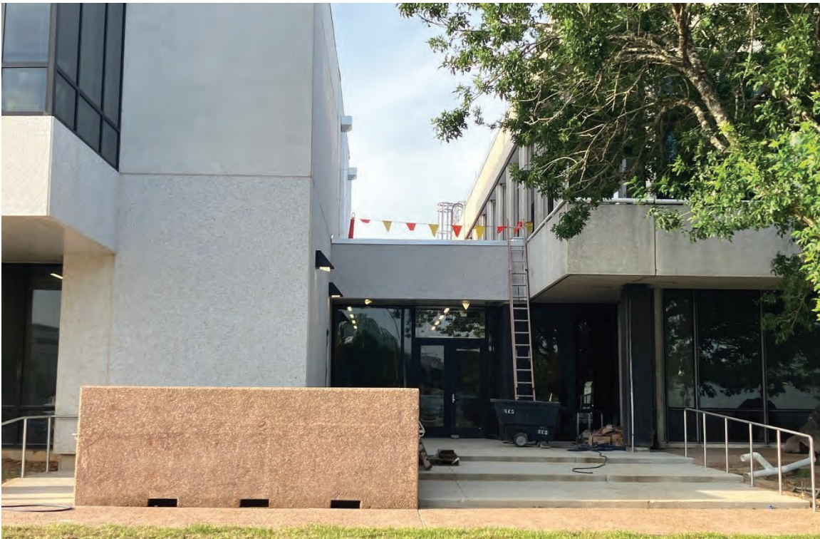
B31X new entrance, nearing construction completion
