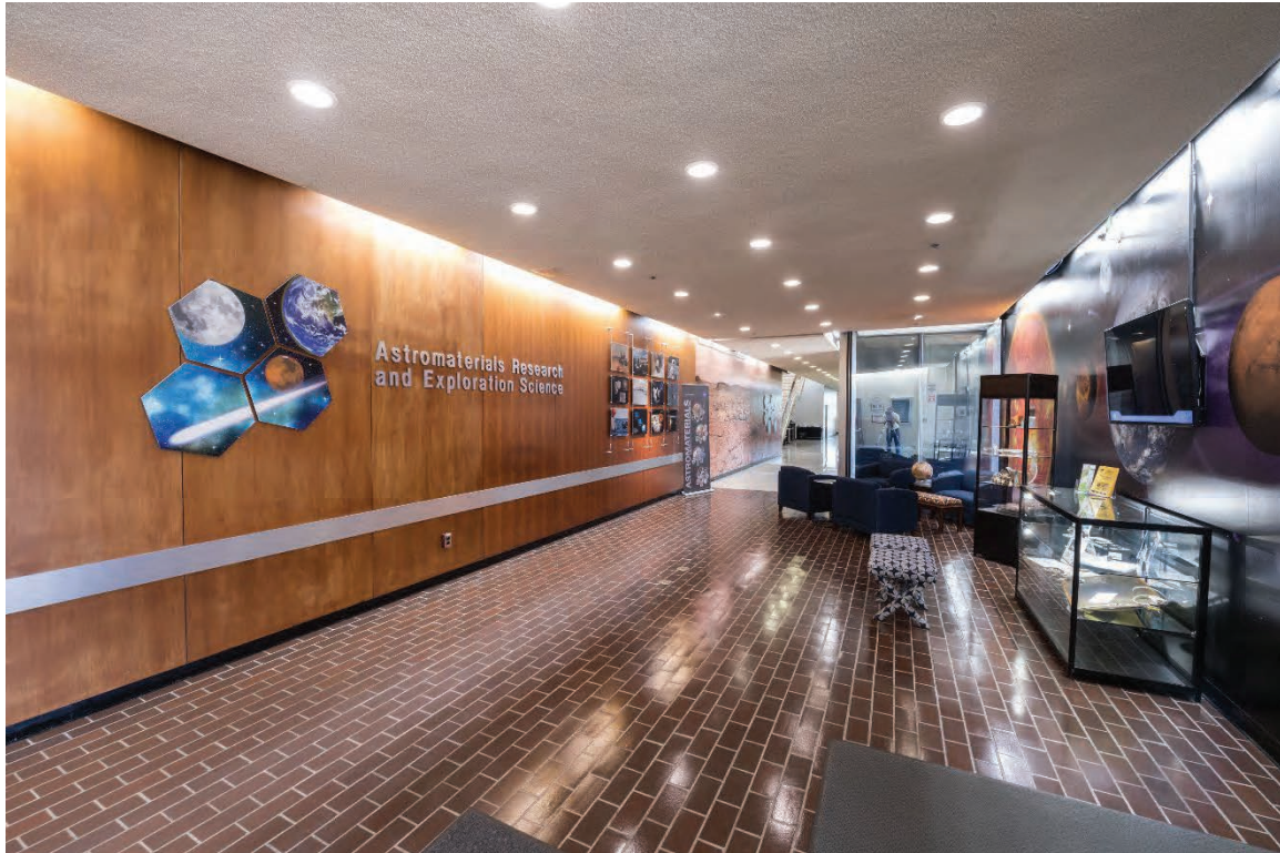
B31 original lobby finishes (brick floor, wood veneer wall) to be preserved
