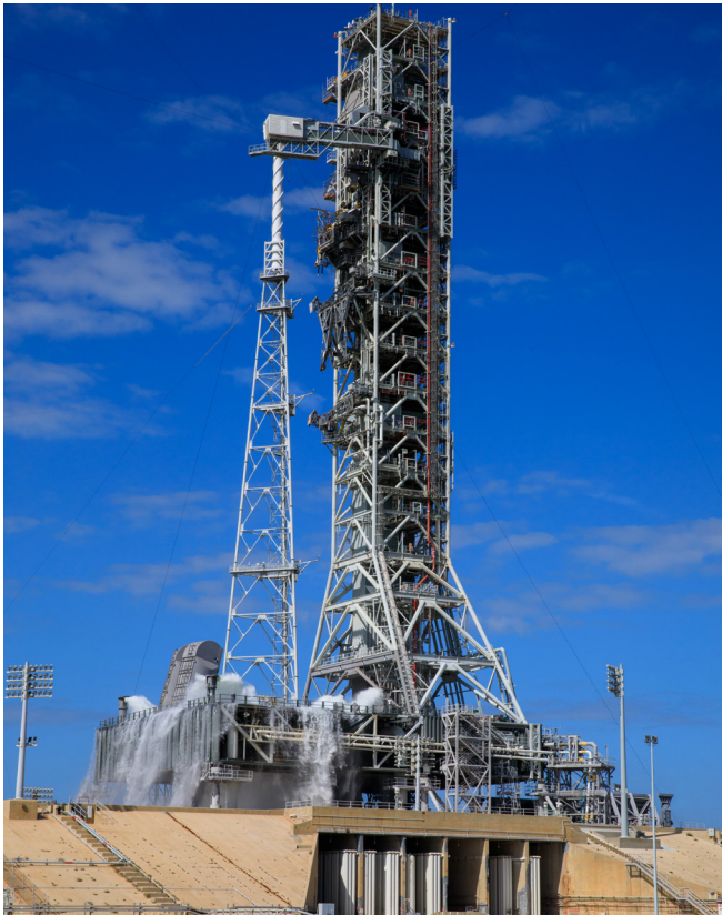
During liftoff, 400,000 gallons of water will rush onto the pad to help protect NASA's SLS (Space Launch System) rocket, Orion spacecraft, mobile launcher, and launch pad from any over pressurization and extreme sound produced during ignition and liftoff. (NASA) ▲
