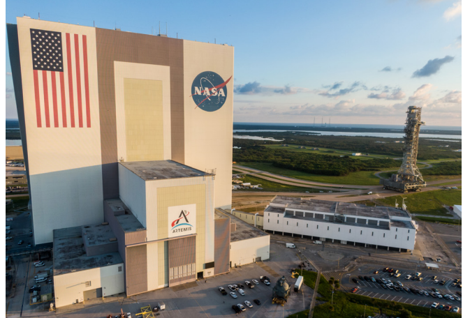
Mobile launcher 1, atop the agency's crawler-transporter 2, moves from Launch Pad 39B, approaching to enter the Vehicle Assembly Building at NASA's Kennedy Space Center on Oct. 3, 2024. (NASA) ▲
