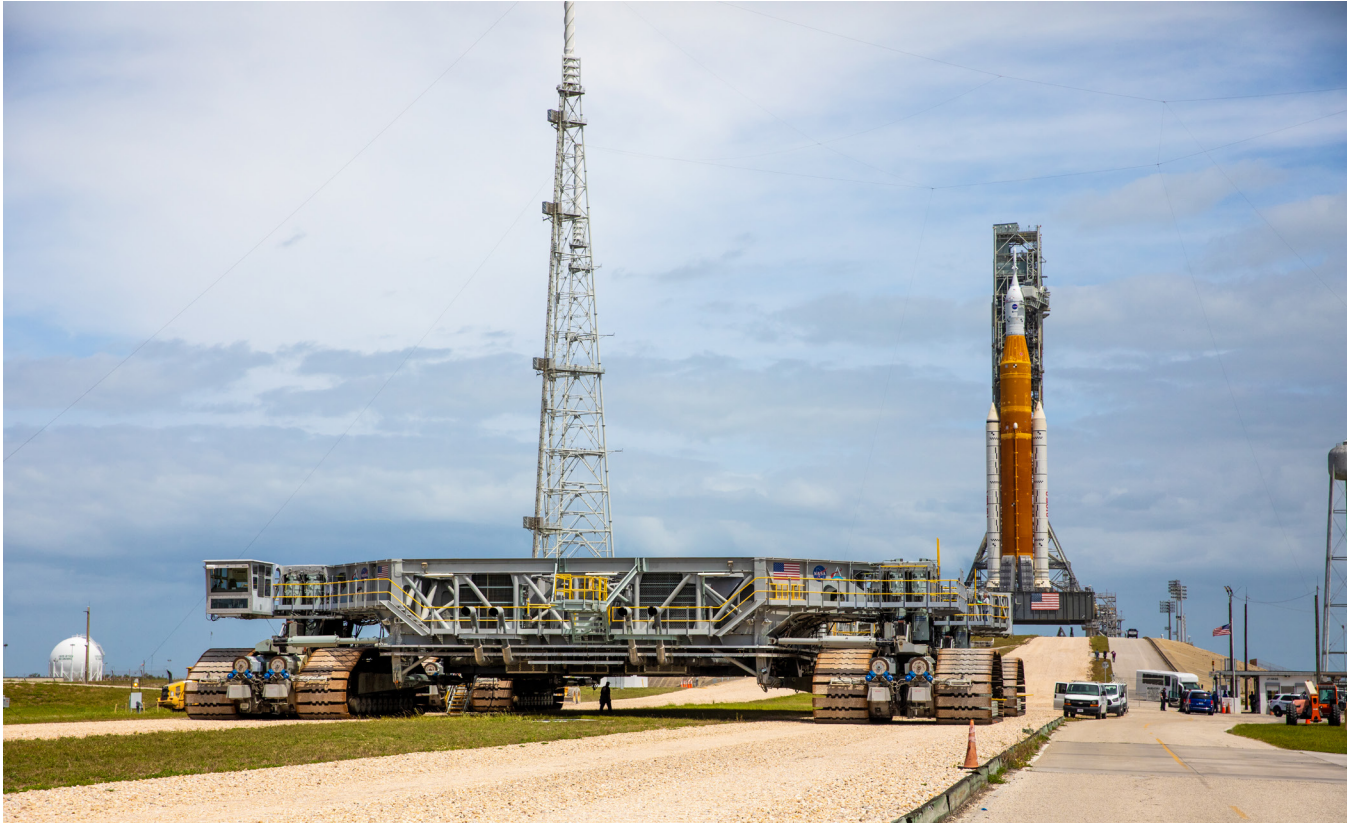
Crawler-transporter 2 makes its way along the crawlerway to Launch Pad 39B. (NASA) ▲
