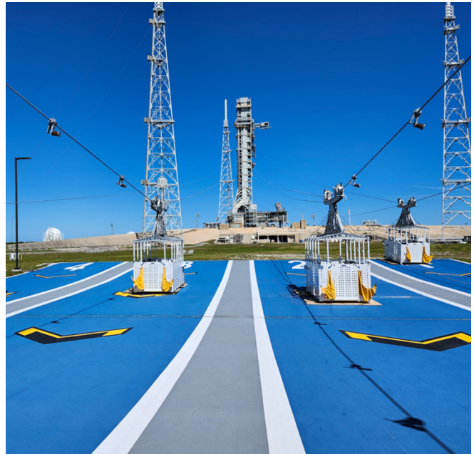
Emergency egress system baskets, attached to the catenary system, rest at the pad terminus site. (NASA) ▲
