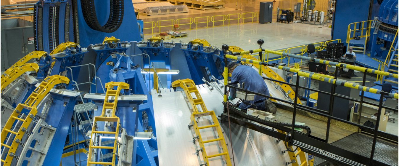
The gore weld tool at Michoud is used to weld domes for the SLS core stage propellant tanks. (NASA) ▲
