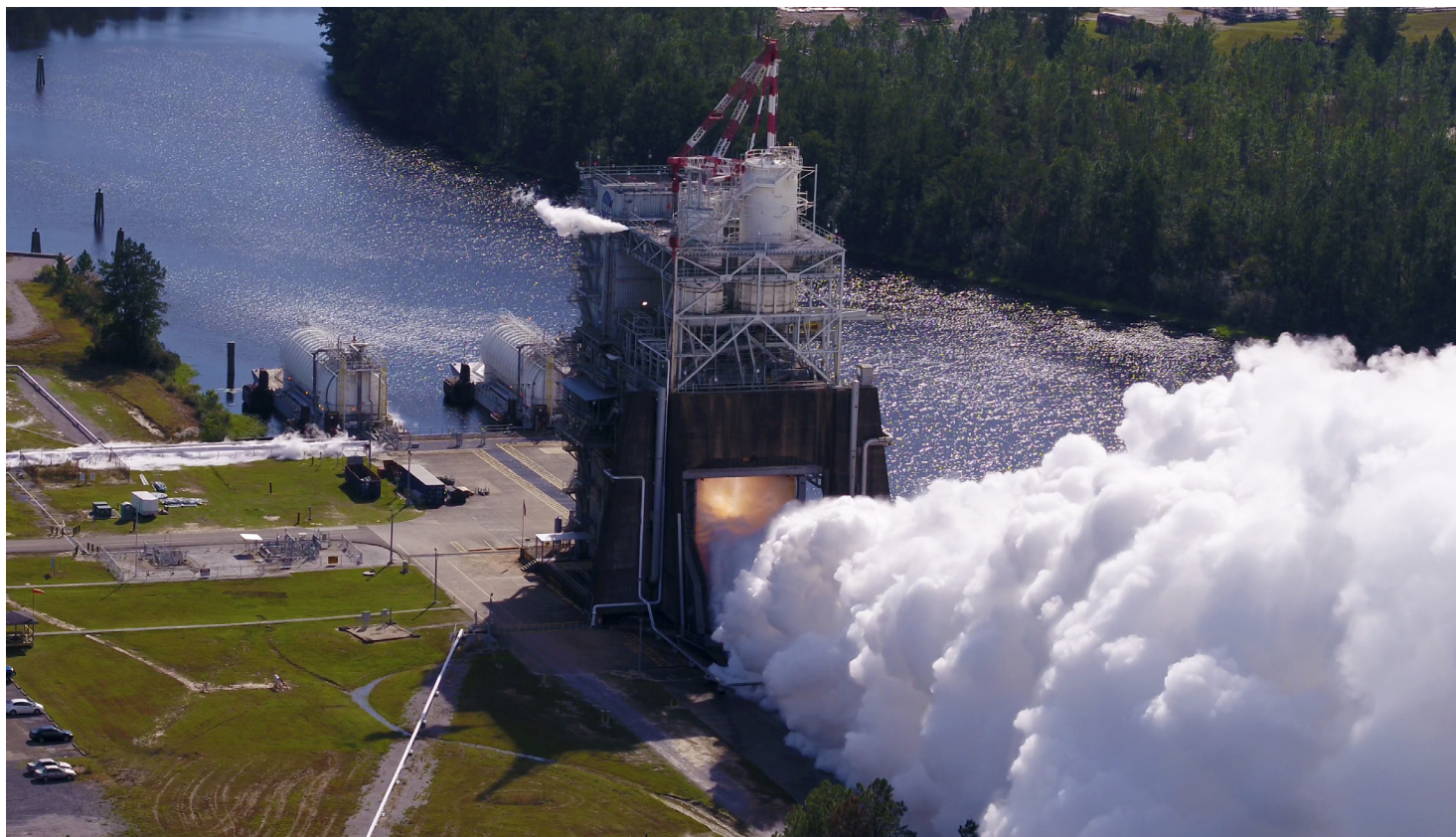
Dedicated ground test RS-25 engines were fired at NASA's Stennis Space Center in Bay St. Louis, Mississippi, to qualify engines to specific SLS operating conditions.
