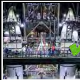
BOOSTER STACKING COMPLETE
