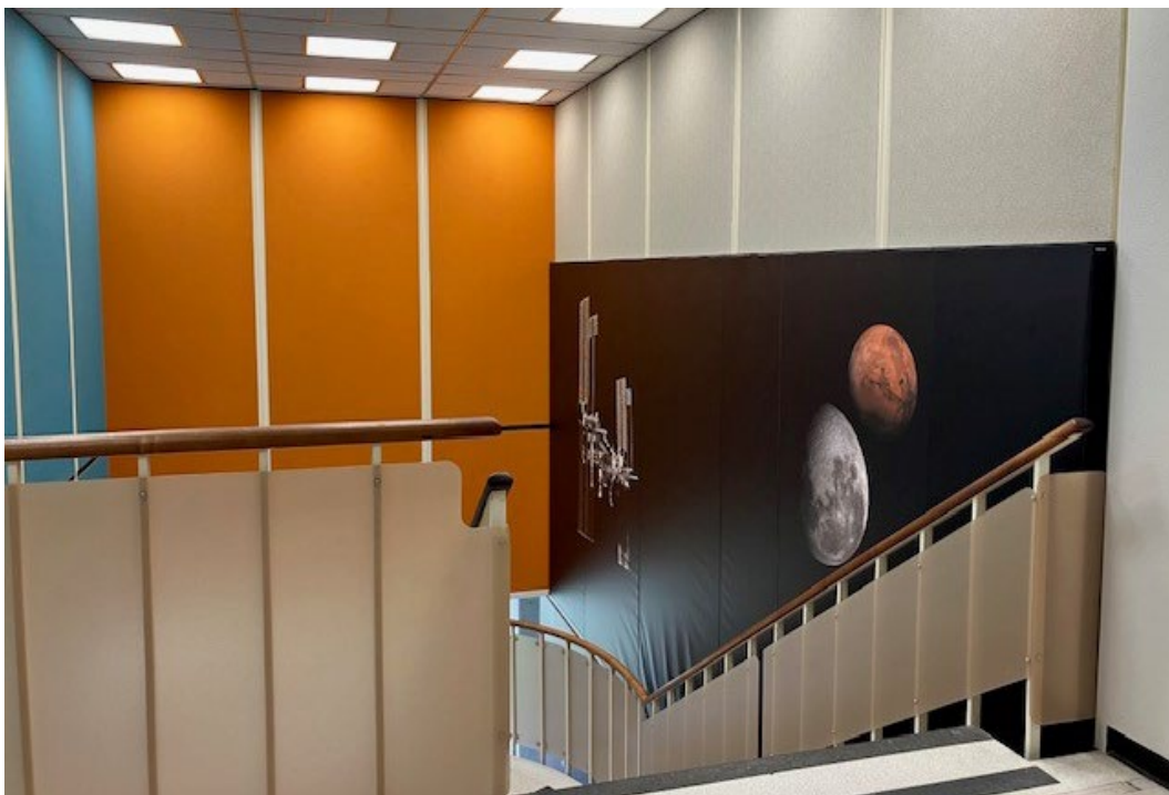
Original staircase; original second floor blue, orange, and gray vinyl wall coverings; and non-original graphic wall covering
