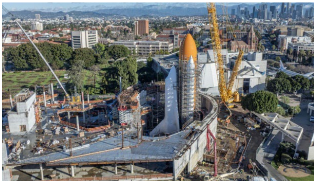
Using flight hardware in the display, the Center was able to use NASA engineering models to validate the seismic capacity of the stacked components. Photo Credit: California Science Center
