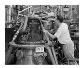
20,000 lb engine being tested in relation with combustion oscillation studies. (Large photo)
