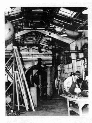
A permanent fixture in the "D" Site Turbine Rig are these dynamatics. Mounted on bed plate, they act as electrical brakes in the overall job of checking the thrust developed by the turbines. Formerly used in Engine Research Building at Lewis, the dynamatics were overhauled and taken to Plum Brook. Ted A. Klonk is seen standing by the dynamatics.
