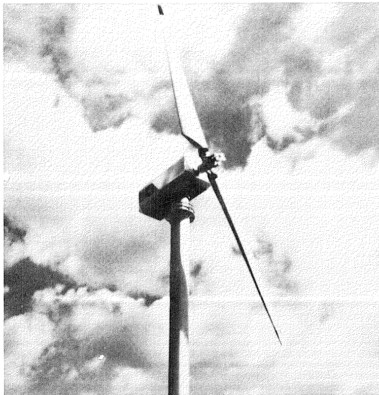
Figure 5. - WTS-4 4000 kW wind turbine.
