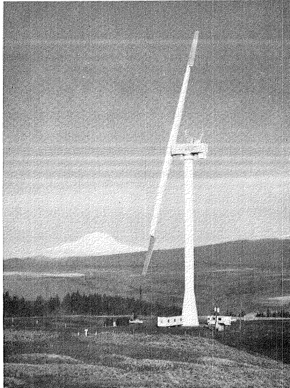
Figure 4. - Mod-2 2500 kW wind turbine.
