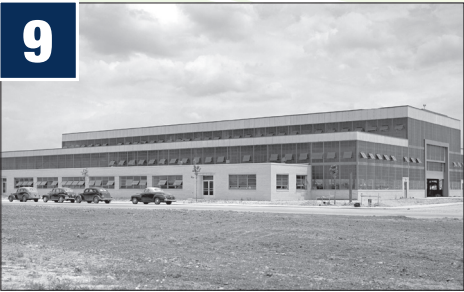
Fabrication Shop (today, Manufacturing Facility)
