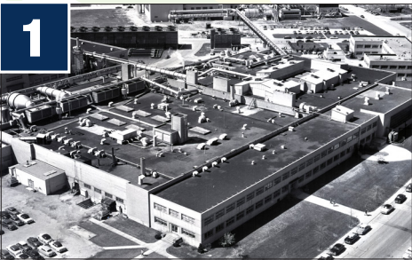
Engine Research Building (ERB)
