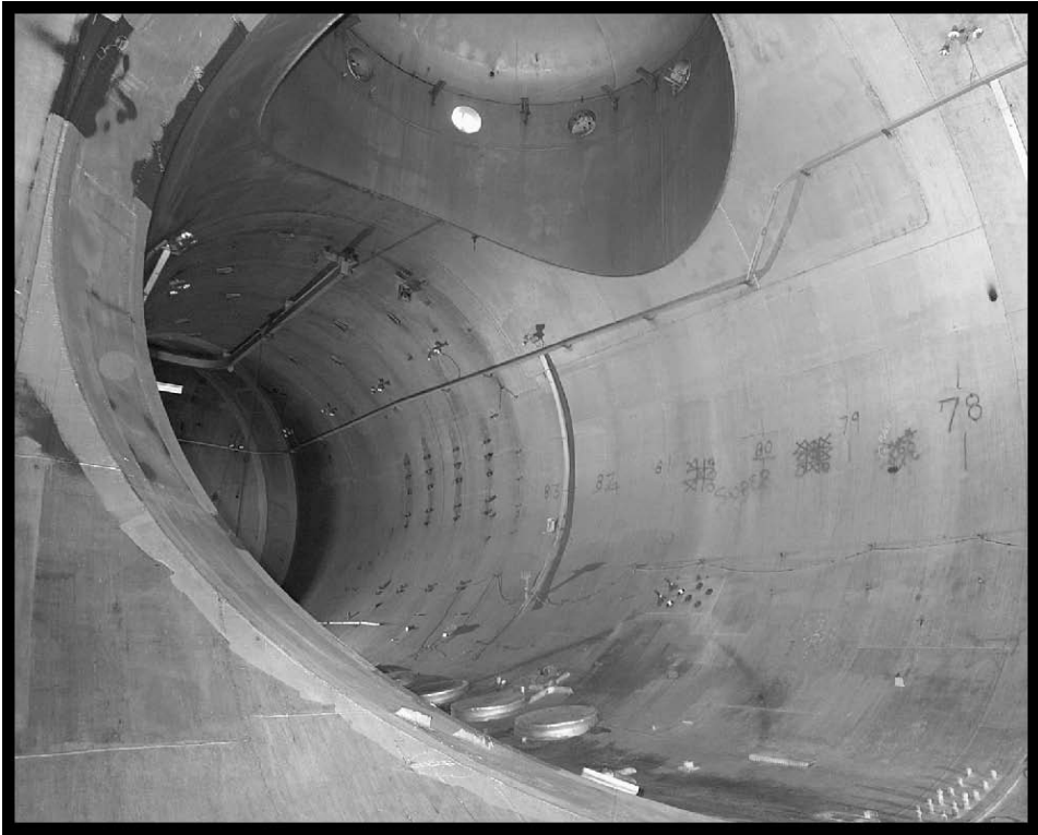
Figure 6.—Interior of SPC No. 1, 2005 (OH_Cuyahoga_Space-Power-Chambers_006).
