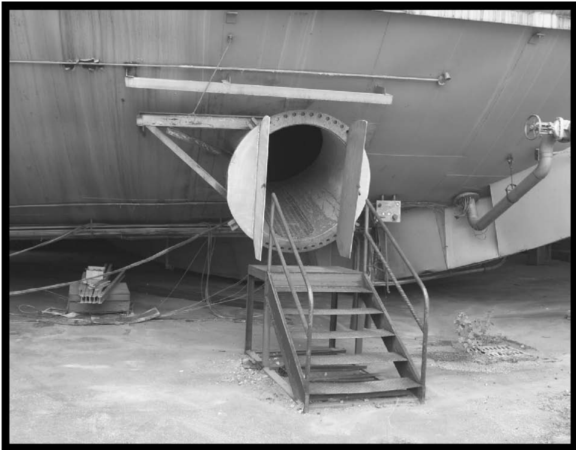
Figure 79.—Interior and exterior of the access door built into the north wall of SPC No. 2, 2005 (OH_Cuyahoga_Space-Power-Chambers_079).
