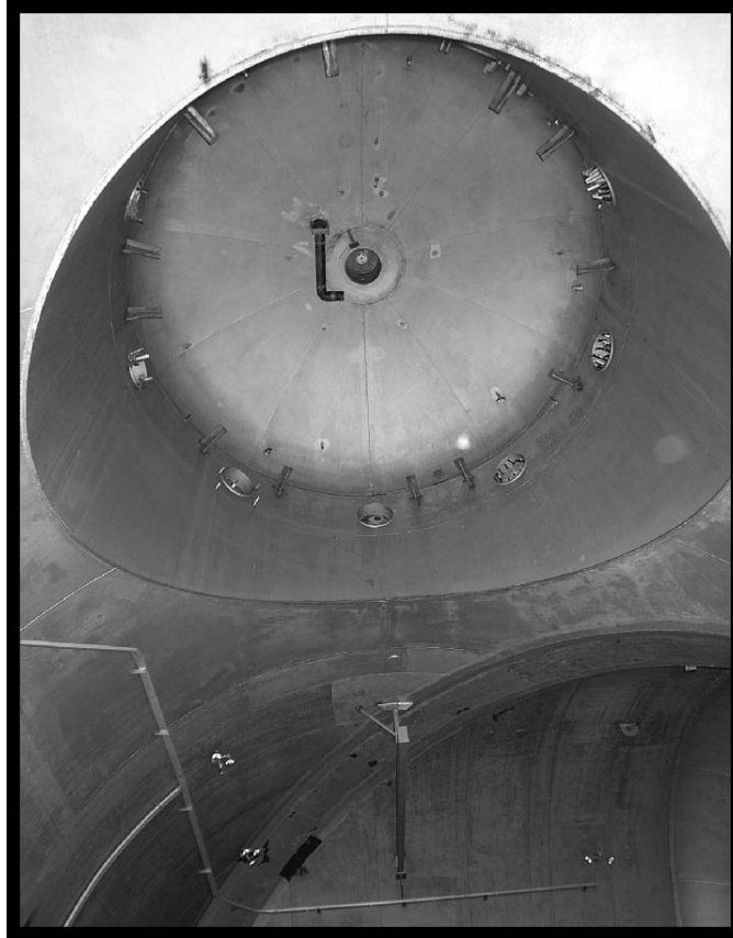
Figure 50.—SPC No. 1 dome and lid (viewed from inside the chamber), 2005 (OH_Cuyahoga_Space-Power-Chambers_050).
