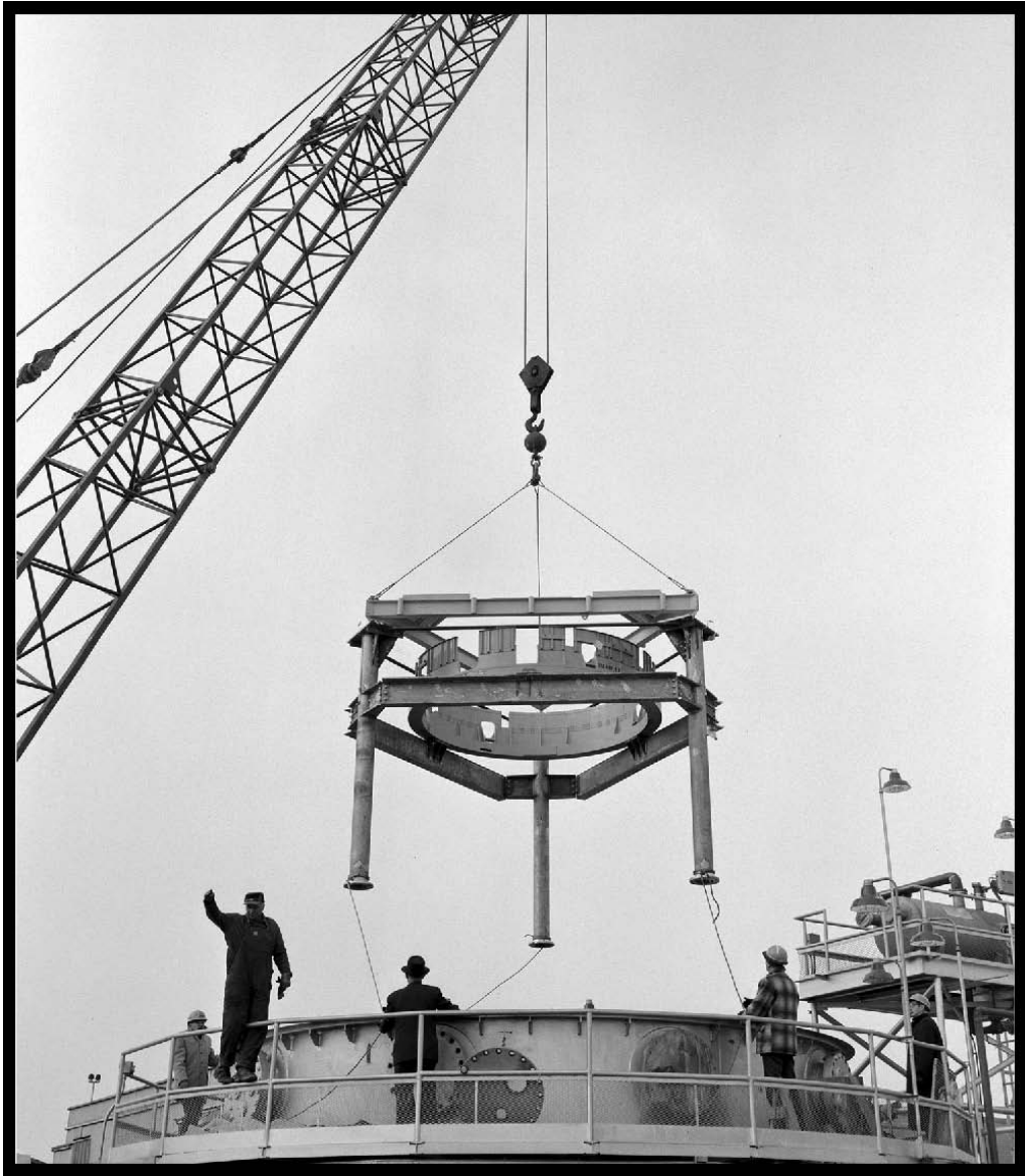
Figure 67.—Stand that supported the Centaur rocket being lifted into SPC No. 1, 1964 (OH_Cuyahoga_Space-Power-Chambers_067).
