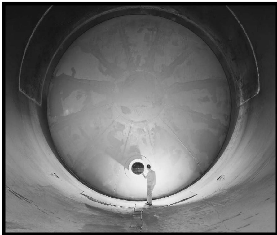
Figure 16.—Bulkhead installed in the southeast corner of the tunnel (viewed from the west), 1962 (OH_Cuyahoga_Space-Power-Chambers_016).
