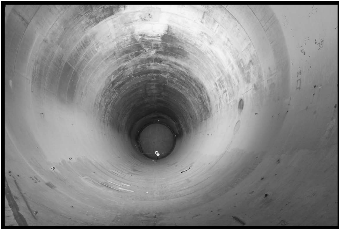
Figure 84.—South leg of SPC No. 2 (viewed from the west), 2007 (OH_Cuyahoga_Space-Power-Chambers_084).
