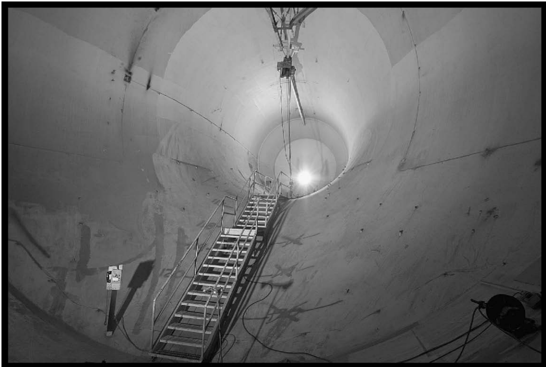
Figure 82.—Throat section of SPC No. 2, showing steps and a telephone in the foreground (viewed from the west), 2007 (OH_Cuyahoga_Space-Power-Chambers_082).
