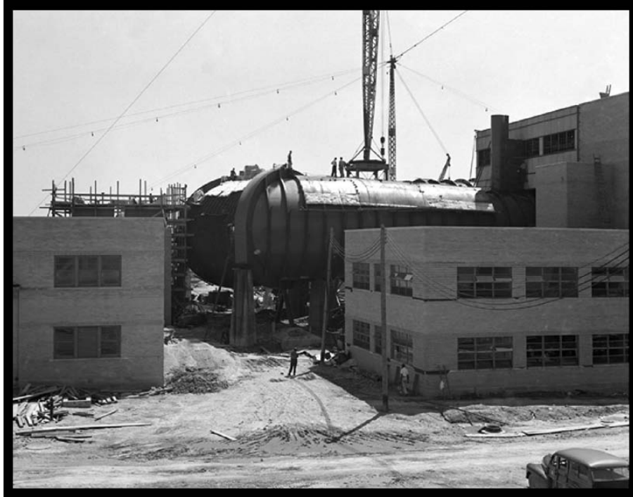
Figure 11.—Original construction of the east leg of the AWT and future SPC No. 1, 1943 (OH_Cuyahoga_Space-Power-Chambers_011).
