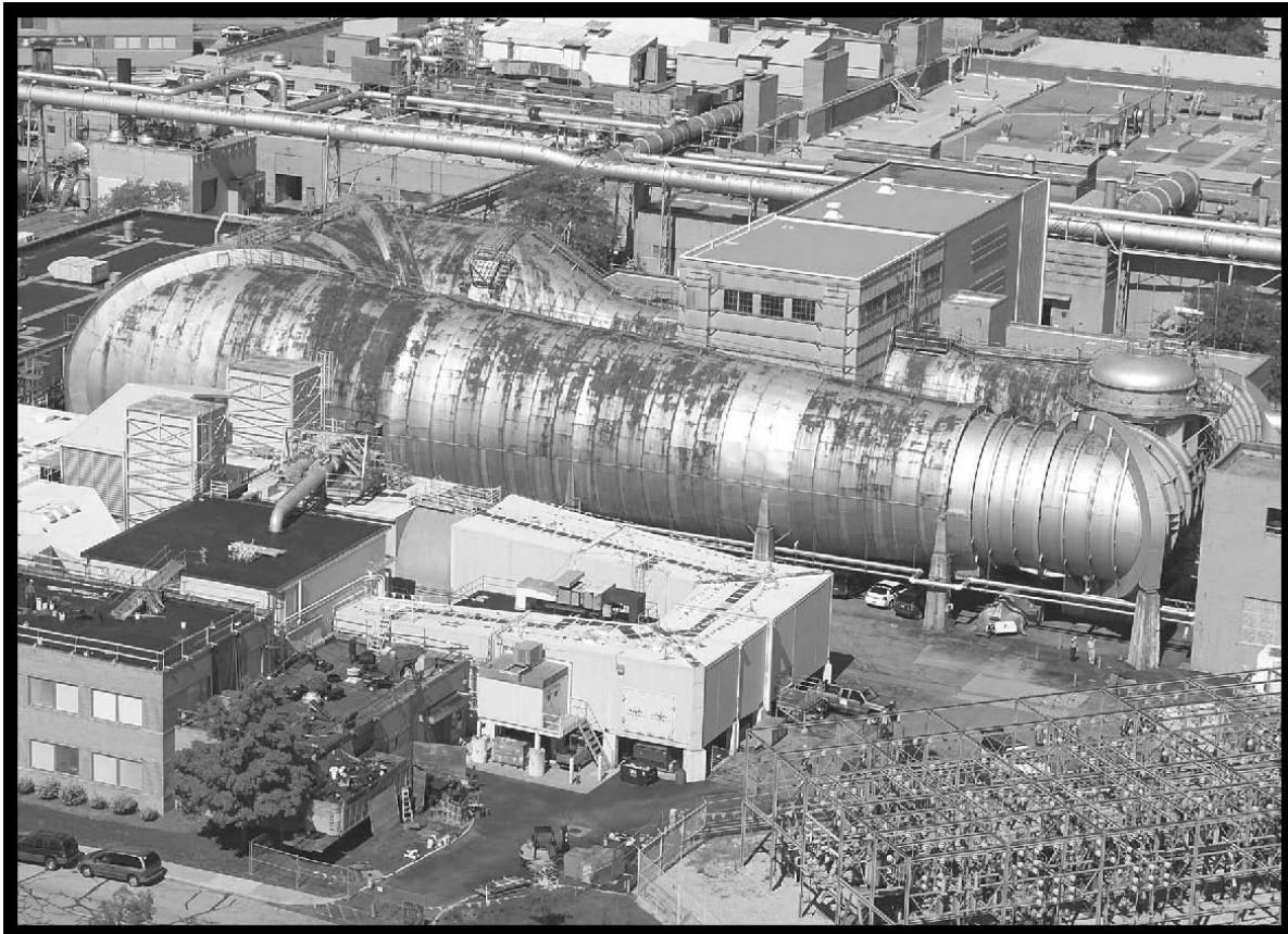
Figure 40.—SPC complex in the former AWT (viewed from the south), 2005 (OH_Cuyahoga_Space-Power-Chambers_040).
