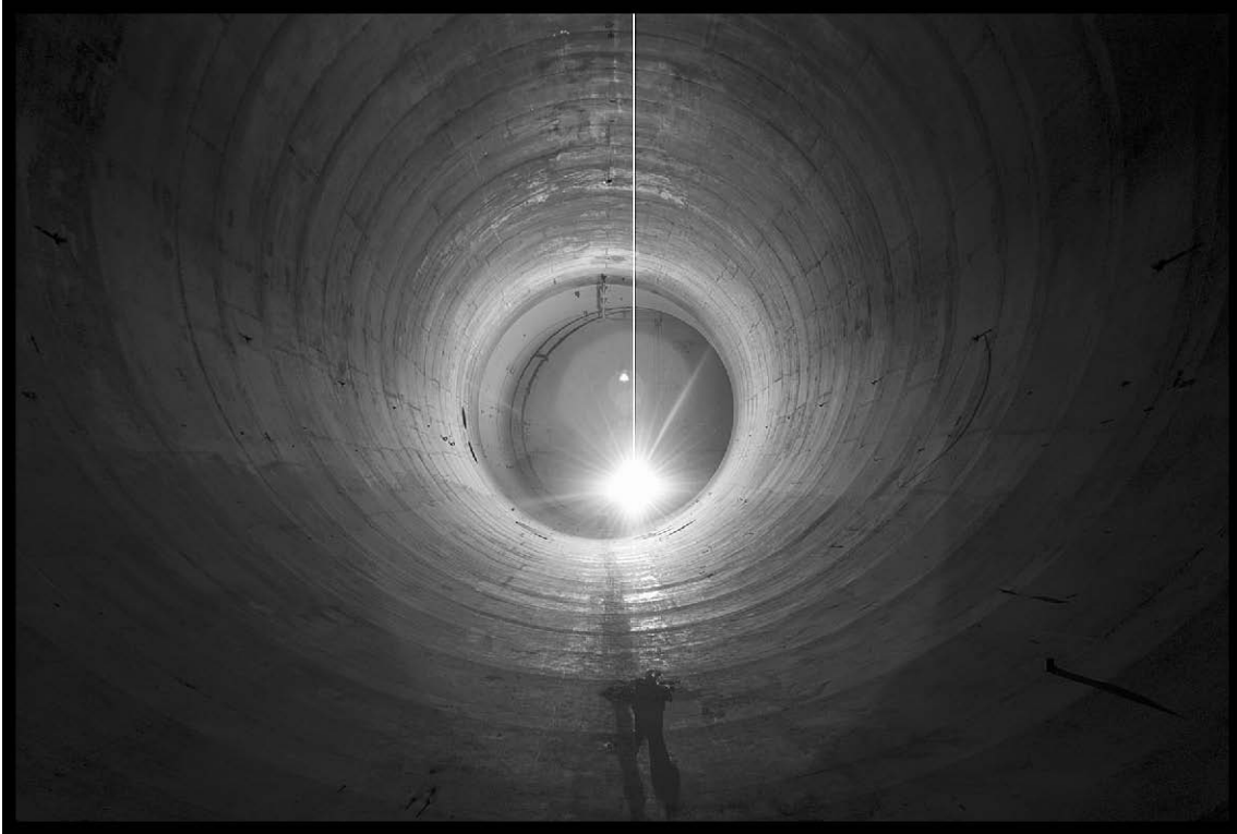
Figure 83.—South leg of SPC No. 2 (viewed from the east), 2007 (OH_Cuyahoga_Space-Power-Chambers_083).
