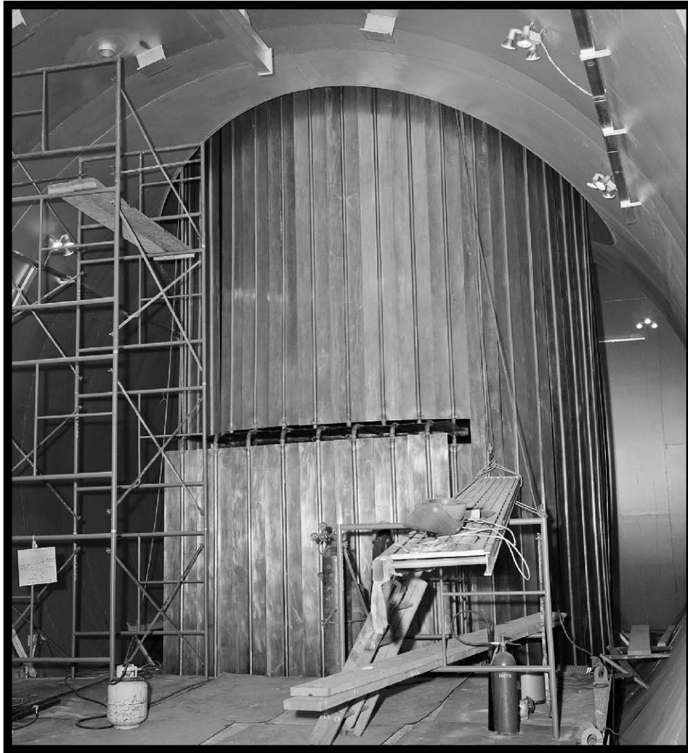
Figure 34.—Nitrogen-filled cold wall (40'-0" high and 20'-0" in diameter) assembled around the Centaur in SPC No. 1, 1963 (OH_Cuyahoga_Space-Power-Chambers_034).
