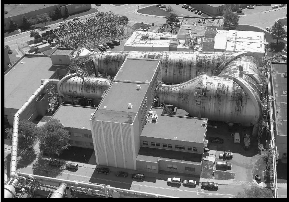
Figure 1.—SPC with SPC No. 1 to the left and SPC No. 2 occupying the rest of the tunnel, 2005 (OH_Cuyahoga_Space-Power-Chambers_001).
