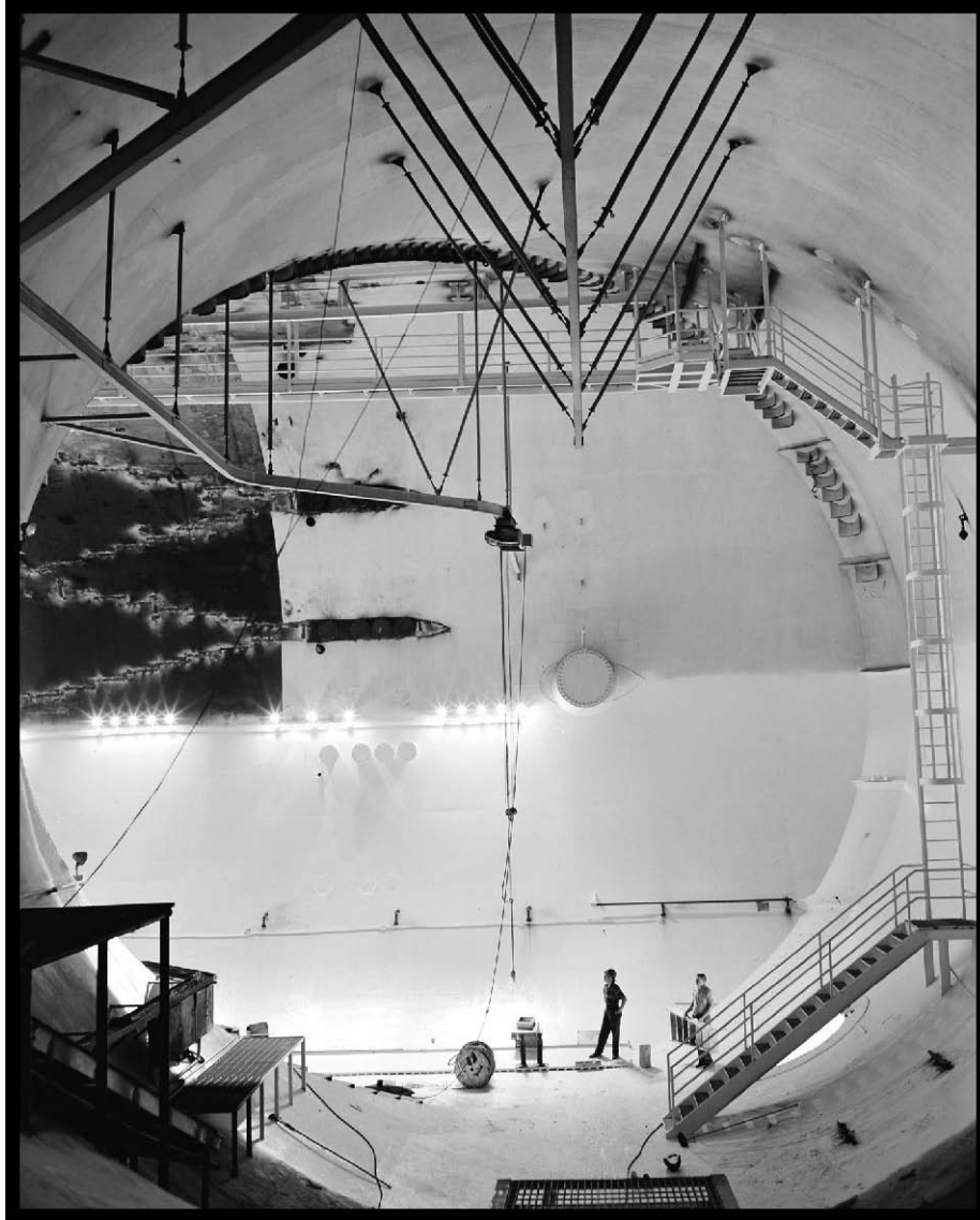
Figure 80.—Throat section of SPC No. 2 showing overhead crane and catwalk (viewed from the east), 1963 (OH_Cuyahoga_Space-Power-Chambers_080).
