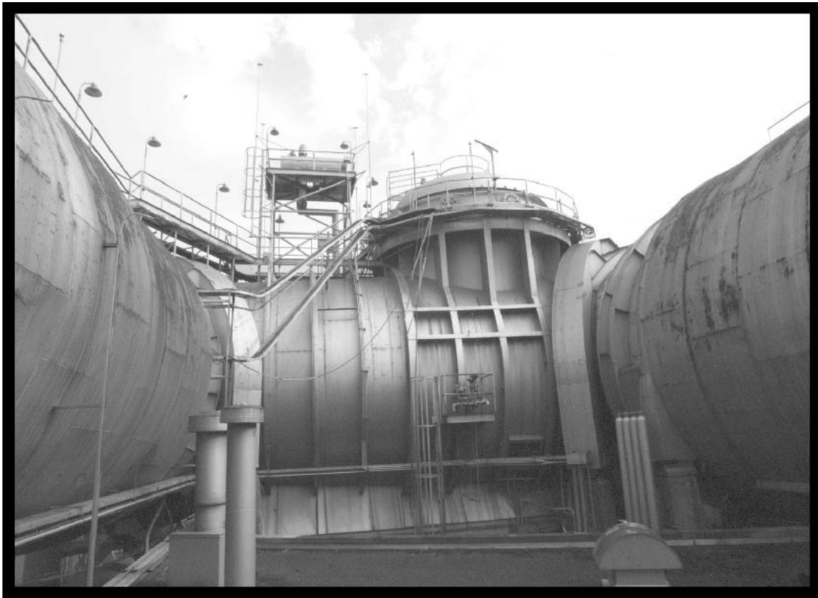
Figure 42.—SPC No. 1 extension and dome (viewed from the west), 2005 (OH_Cuyahoga_Space-Power-Chambers_042).
