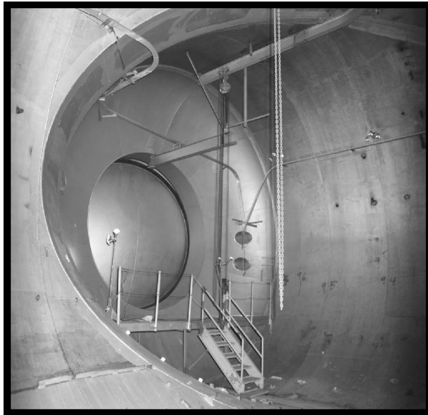
Figure 57.—Platform inside SPC No. 1 that provided access to the doorway in the bulkhead, 2005 (OH_Cuyahoga_Space-Power-Chambers_057).
