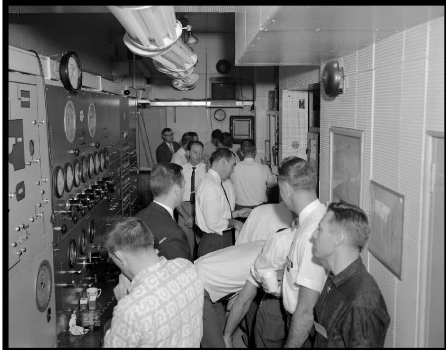
Figure 98.—Interior of SPC No. 2 control room with the control panel on the left (viewed from the east), 1963 (OH_Cuyahoga_Space-Power-Chambers_098).
