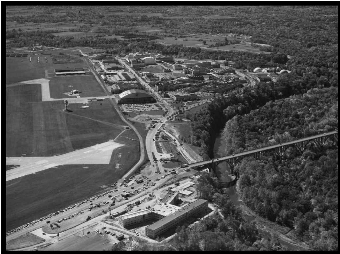
Figure 10.—NASA Lewis, showing the Cleveland Municipal Airport (left), the Rocky River valley (right), and the city of North Olmsted (background) (viewed from the northeast), 1963 (OH_Cuyahoga_Space-Power-Chambers_010).
