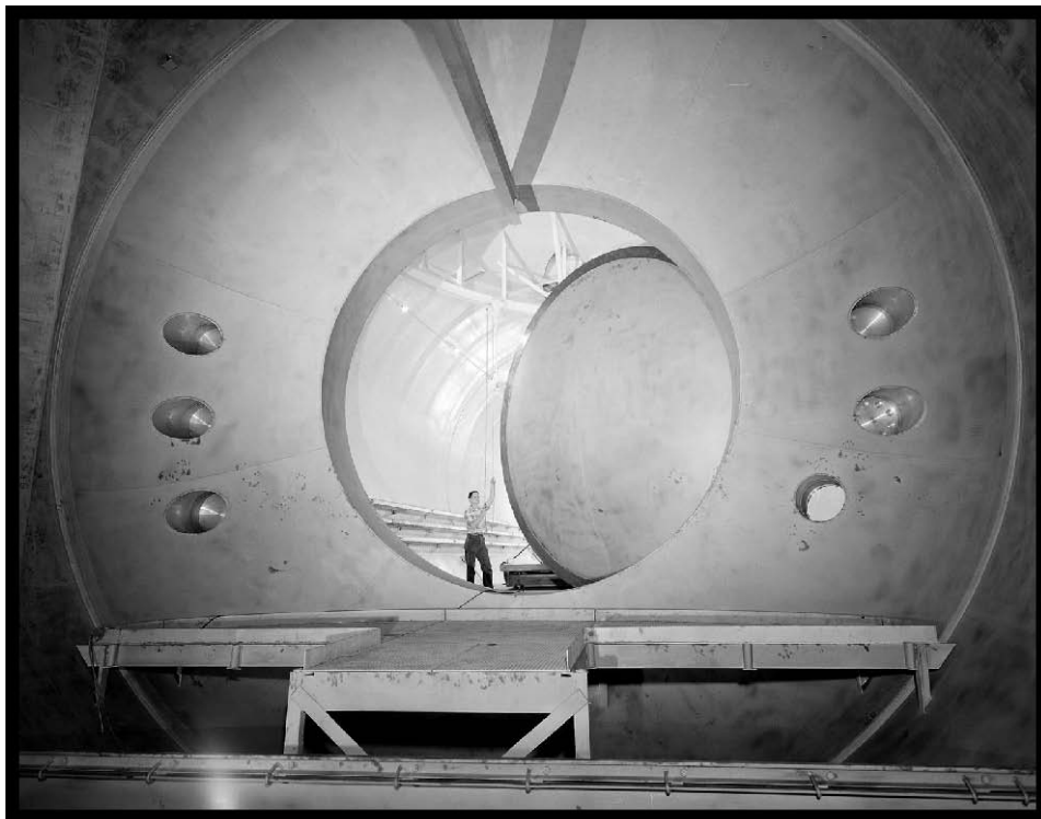
Figure 53.—Inside SPC No. 1 bulkhead with a swinging door in the center and ports on the sides (viewed from the east), 1962 (OH_Cuyahoga_Space-Power-Chambers_053).
