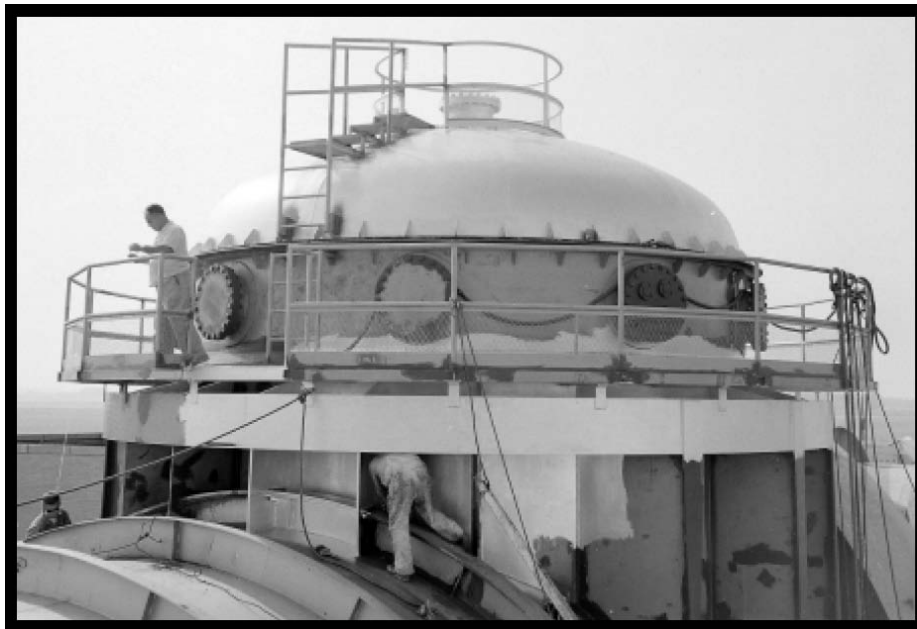
Figure 46.—SPC No. 1 dome showing its base, instrumentation portals, and lid (viewed from the north), 1963 (OH_Cuyahoga_Space-Power-Chambers_046).
