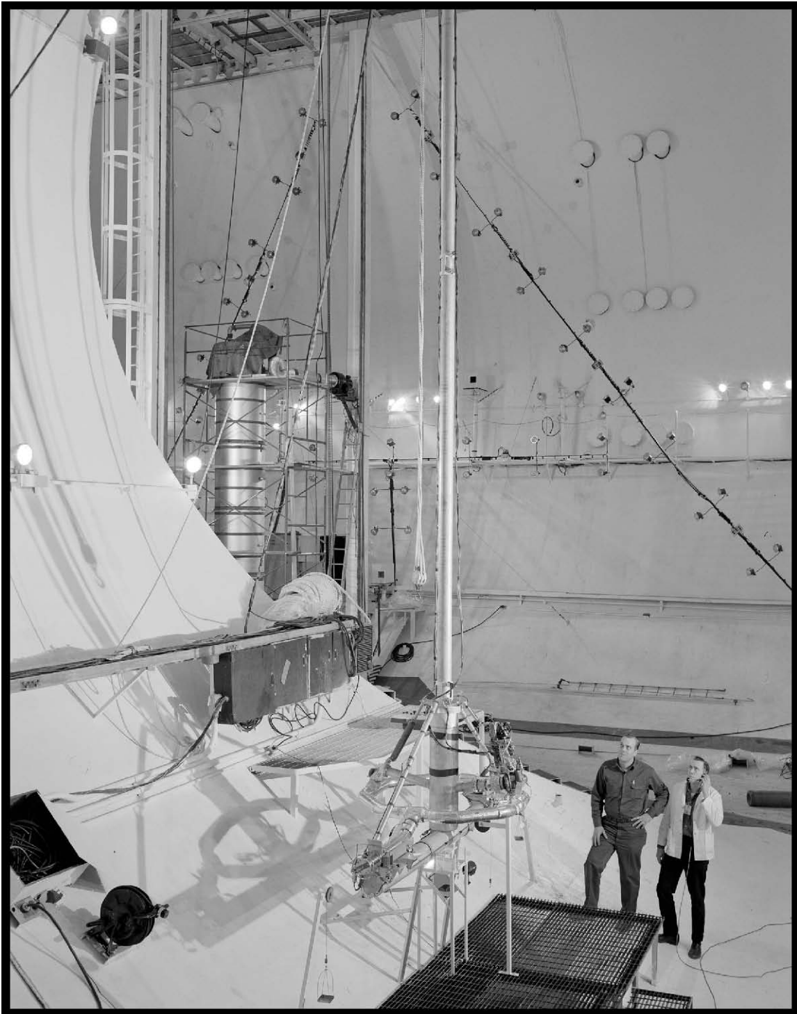
Figure 92.—Equipment mounted to the interior wall near the throat section, 1965 (OH_Cuyahoga_Space-Power-Chambers_092).
