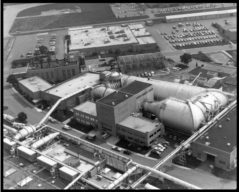
Figure 5.—SPC with Solar Power Laboratory (left), Shop and Office Building (center), and Refrigeration Building (right), 1979 (OH_Cuyahoga_Space-Power-Chambers_005).
