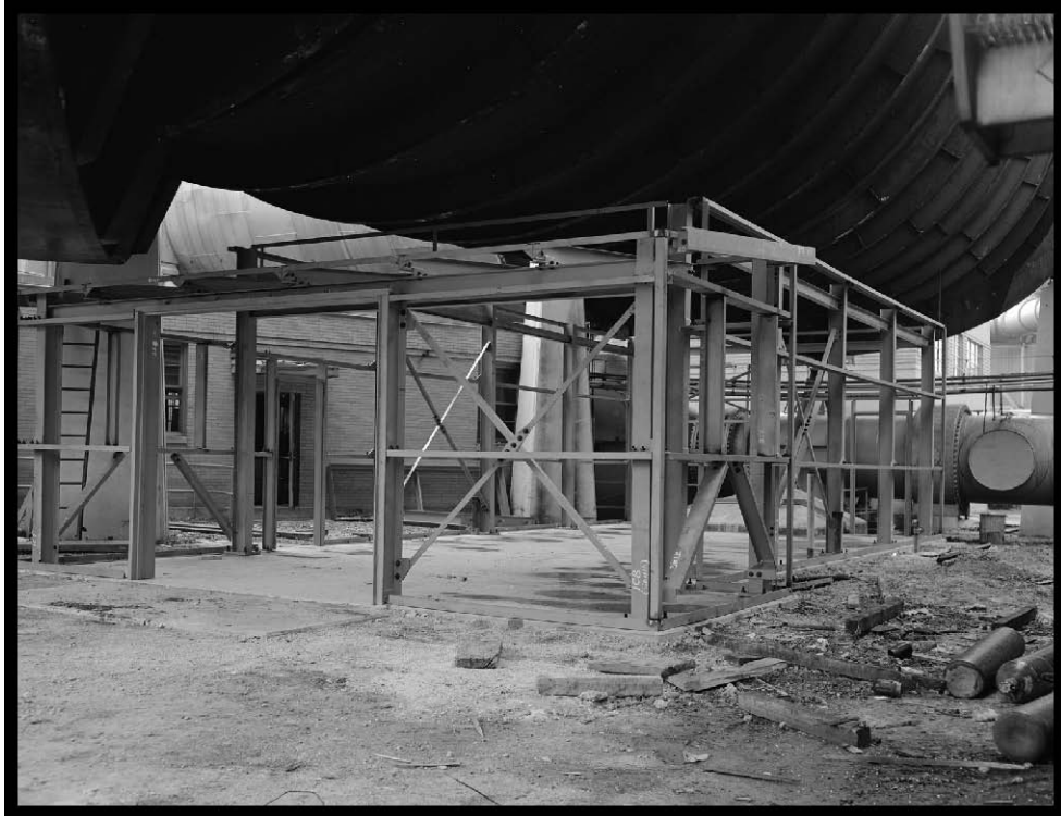
Figure 64.—Construction of Vacuum Pump House beneath SPC No. 1, 1961 (OH_Cuyahoga_Space-Power-Chambers_064).
