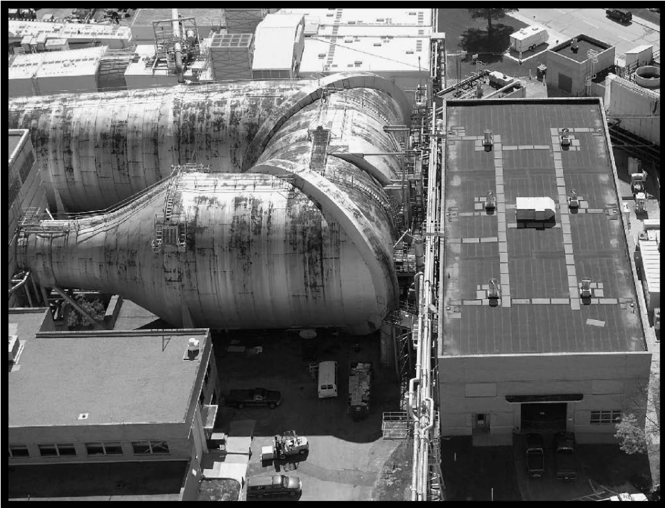
Figure 73.—Exterior of SPC No. 2 (aerial view from the north), 2005 (OH_Cuyahoga_Space-Power-Chambers_073).
