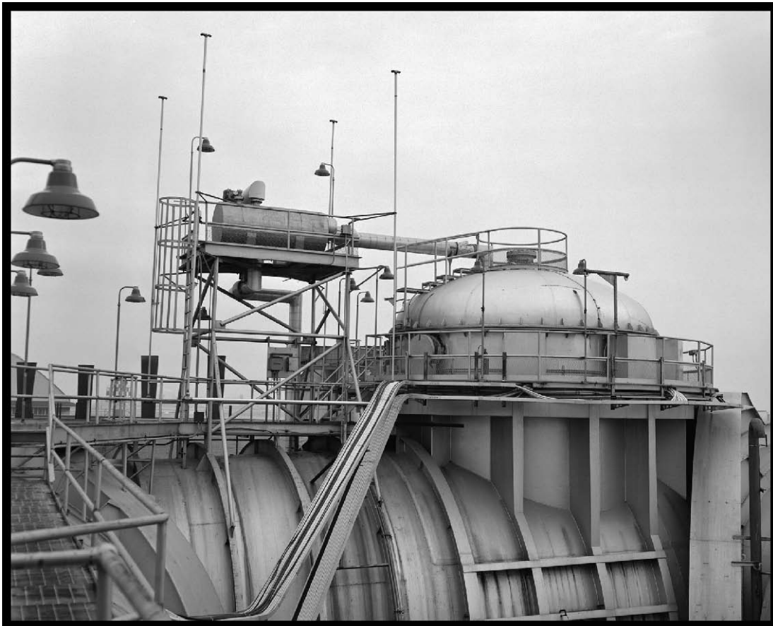
Figure 68.—The nitrogen separation tank setup to left of the dome supplied the cold wall inside with coolant, 1967 (OH_Cuyahoga_Space-Power-Chambers_068).
