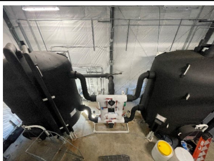
Granulated Activated Carbon (GAC) treatment units at the WFF for the removal of PFAS contamination from the Town of Chincoteague water supply.
