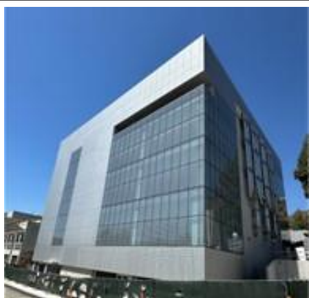
NASA's Flight Electronics Integration Facility at JPL consolidates electronic component processing of flight hardware for NASA missions led by JPL.
