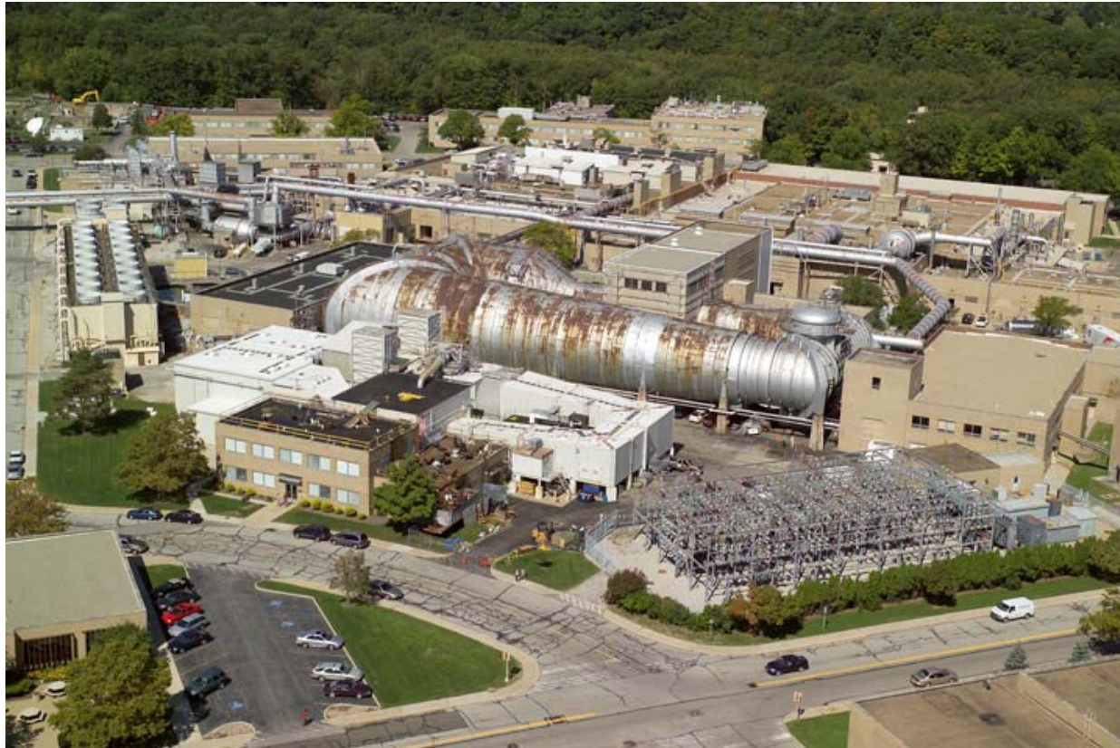
Photograph No. 1 - Altitude Wind Tunnel Viewed from the South with the Icing Research Tunnel and Substation "B" in the Foreground
