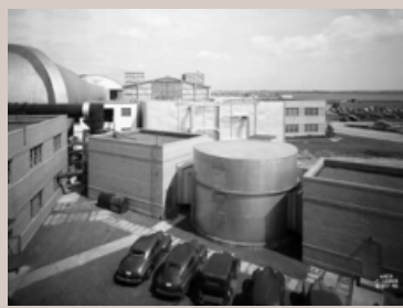
Air Dryer Building
