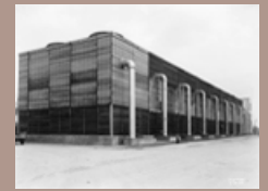
Cooling Tower in 1951
