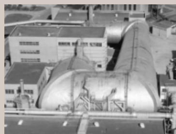
AWT Roof with Walkway
