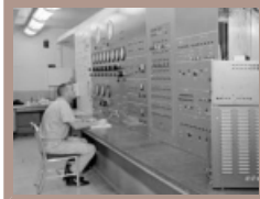
SPC No. 2 Controls
