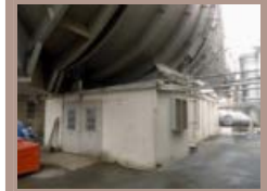
Pump House in 2007
