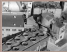
Air Dryer Building
