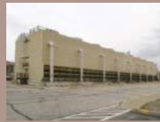
Cooling Tower in 2005
