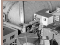
Stack Tunnel Aerial
