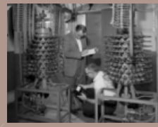
AWT Damper Room
