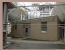
Pump House in 2007
