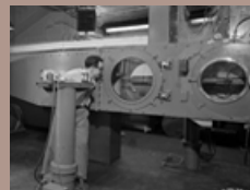
Ramjet in Small Tunnel
