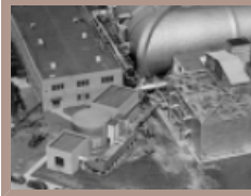
Air Dryer Building
