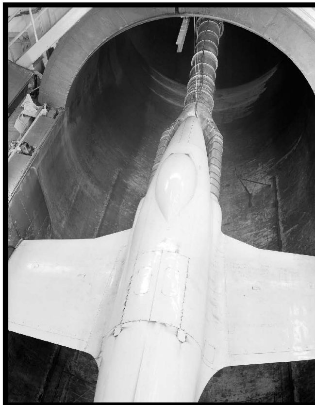
Figure 35.—Bell YP-80 Shooting Star installed in the AWT test section, 1945 (OH_Cuyahoga_Altitude-Wind-Tunnel_036).
