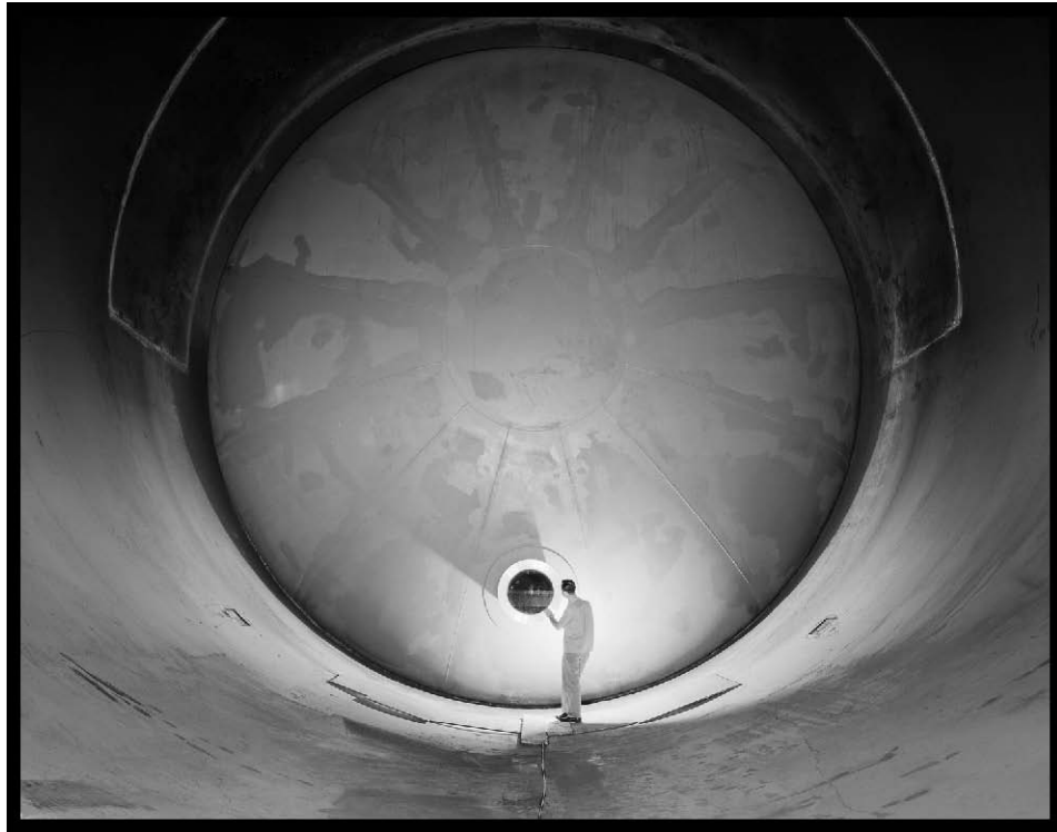
Figure 26.—31'-0"-diameter bulkhead that was added to the southeast corner of the AWT to create the SPC, 1962 (OH_Cuyahoga_Altitude-Wind-Tunnel_027).
