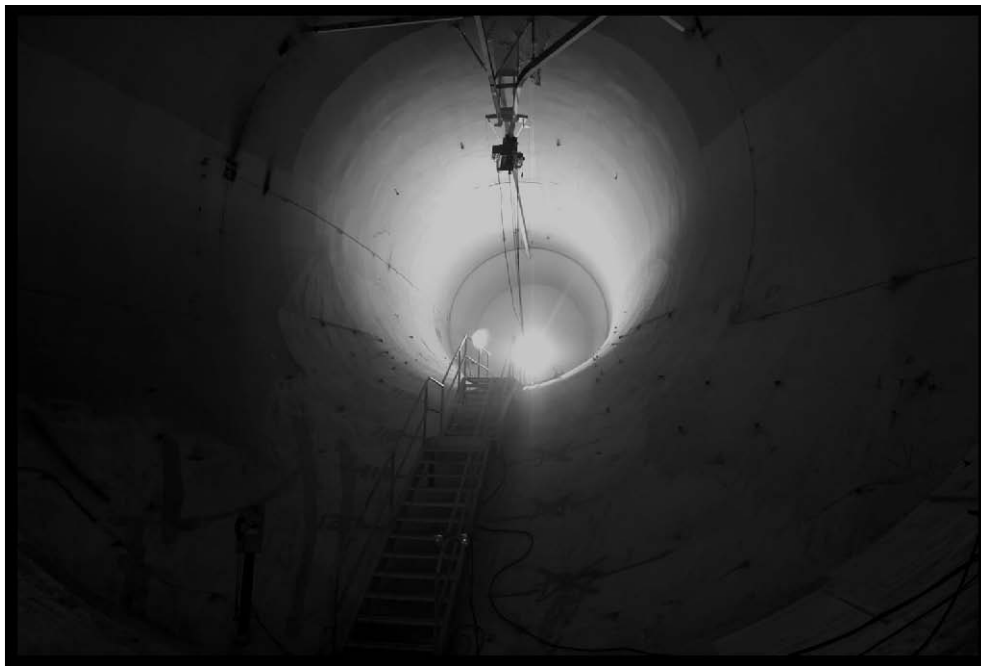
Figure 76.—Throat section of the AWT (viewed from the northwest corner), 2007 (OH_Cuyahoga_Altitude-Wind-Tunnel_077).
