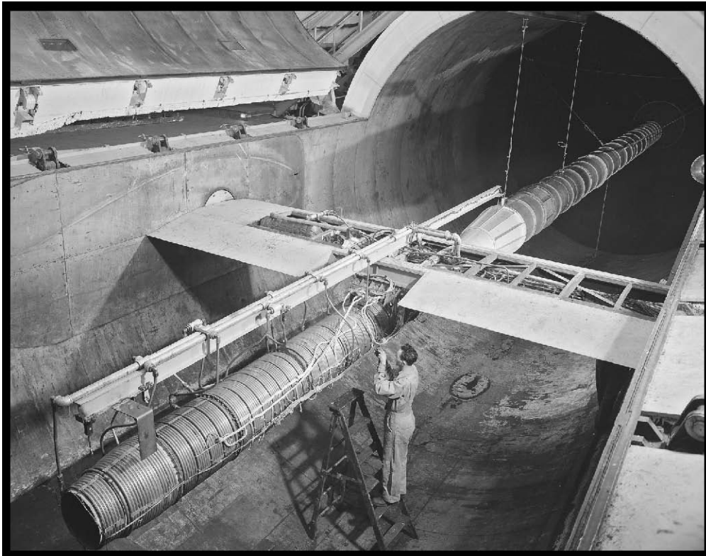
Figure 93.—Makeup air line shown extended into the test section and attached directly to the engine inlet, 1944 (OH_Cuyahoga_Altitude-Wind-Tunnel_094).
