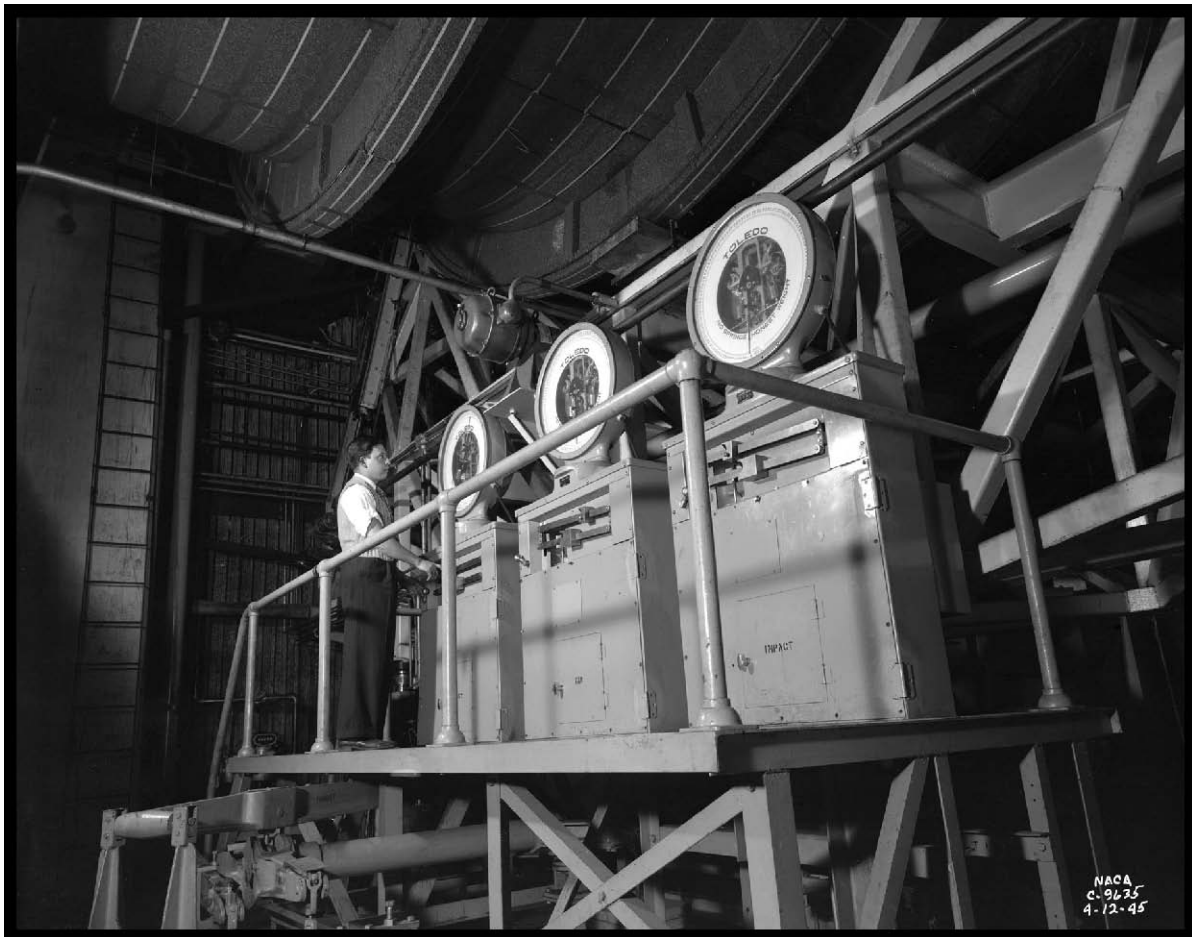
Figure 114.—Toledo scales and balance frame underneath the AWT test section, 1945 (OH_Cuyahoga_Altitude-Wind-Tunnel_115).
