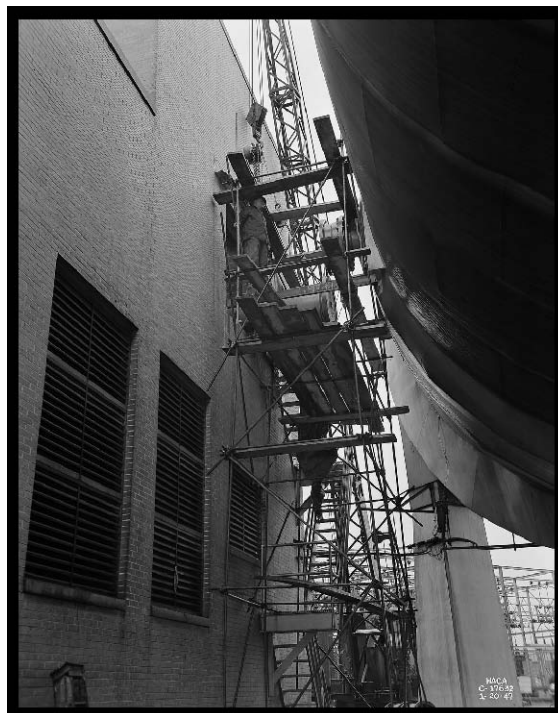
Figure 89.—Drive shaft being installed at the propeller hatch on the southeast corner of the AWT (viewed from the east), 1947 (OH_Cuyahoga_Altitude-Wind-Tunnel_090).
