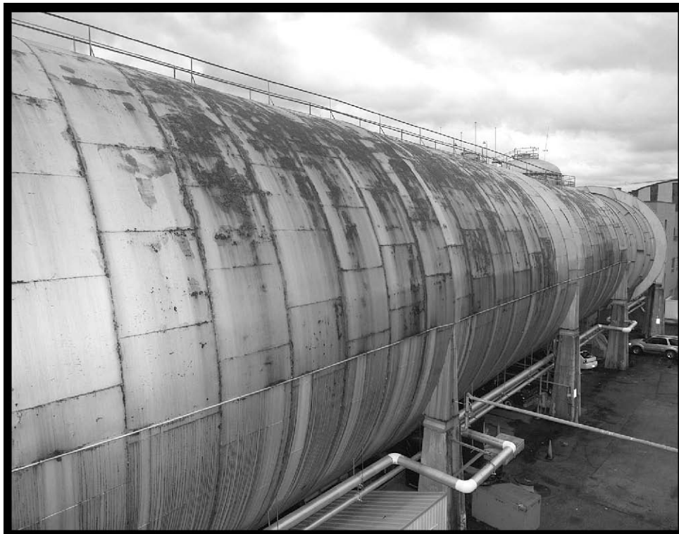
Figure 45.—AWT's south leg (viewed from the west), 2005 (OH_Cuyahoga_Altitude-Wind-Tunnel_046).
