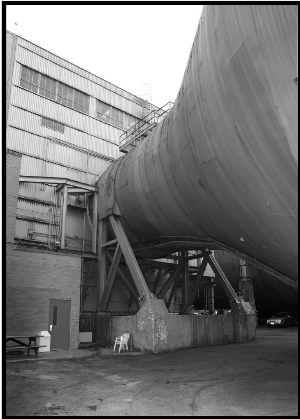
Figure 115.—Balance chamber piers were visible from outside of the test chamber (viewed from the northwest), 2005 (OH_Cuyahoga_Altitude-Wind-Tunnel_116).
