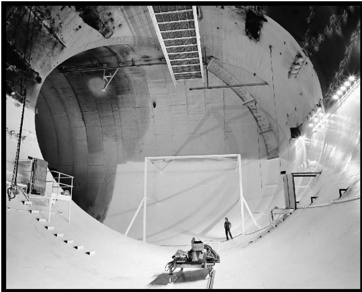
Figure 71.—Wide western leg of the AWT, with the cooling coils and turning vanes removed (viewed from the north), 1963 (OH_Cuyahoga_Altitude-Wind-Tunnel_072).
