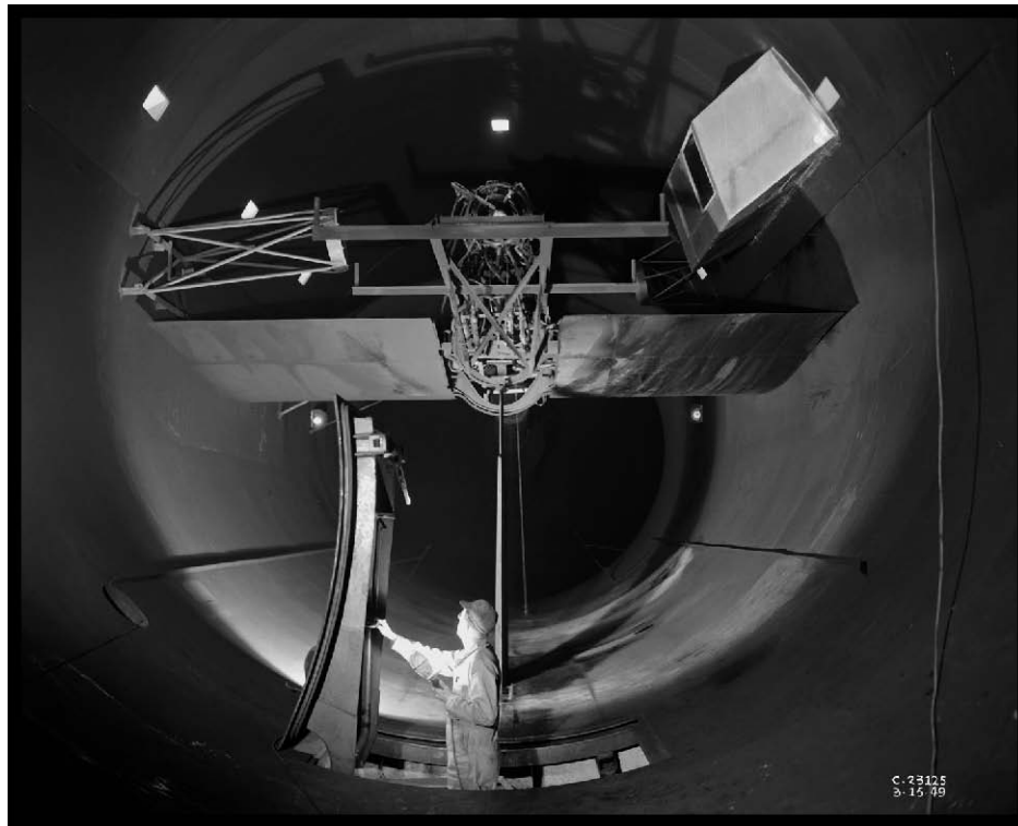
Figure 108.—A technician enters the AWT test section through a doorway in the floor, 1949 (OH_Cuyahoga_Altitude-Wind-Tunnel_109).
