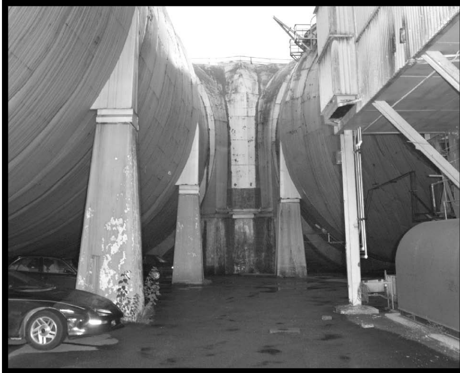
Figure 57.—Inside of the AWT loop showing the pylons and west-end concrete base (viewed from the east), 2005 (OH_Cuyahoga_Altitude-Wind-Tunnel_058).
