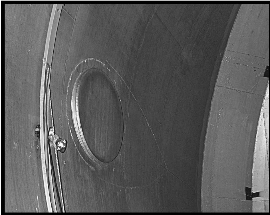
Figure 81.—Sealed penetration where the drive shaft for the AWT's fan was formerly located, 2005 (OH_Cuyahoga_Altitude-Wind-Tunnel_082).
