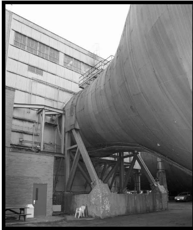
Figure 48.—AWT's throat section as it enters the test chamber (viewed from the northeast), 2005 (OH_Cuyahoga_Altitude-Wind-Tunnel_049).
