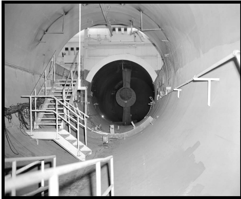
Figure 77.—View from the throat section through the former 20'-0"-diameter test section with the air scoop at the far end, 1961 (OH_Cuyahoga_Altitude-Wind-Tunnel_078).
