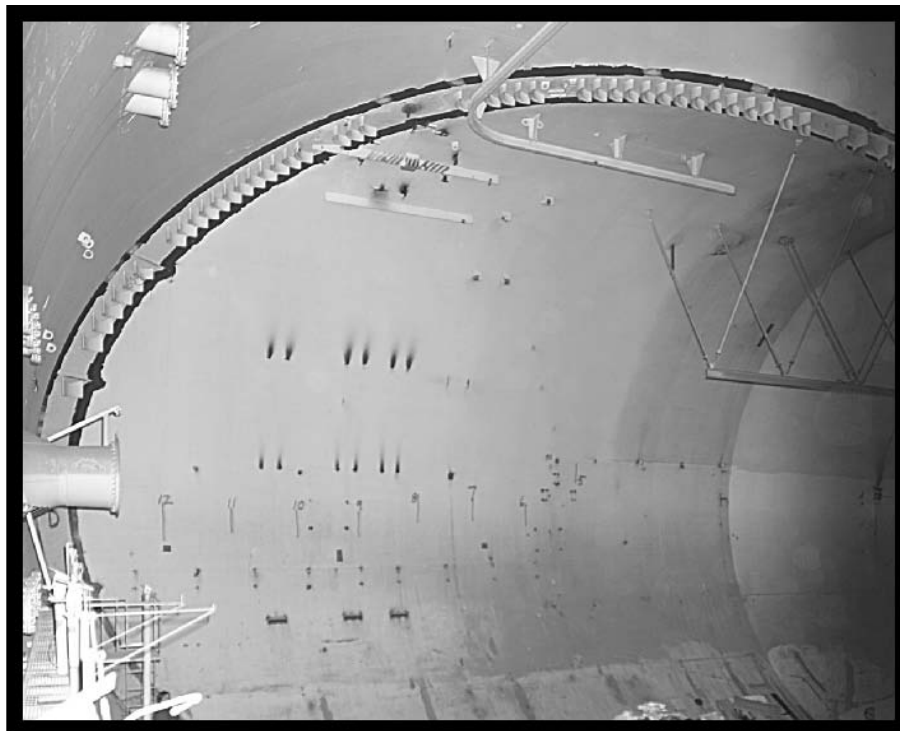
Figure 91.—Fixtures that held a panel of turning vanes in the northwest corner of the AWT, 2005 (OH_Cuyahoga_Altitude-Wind-Tunnel_092).
