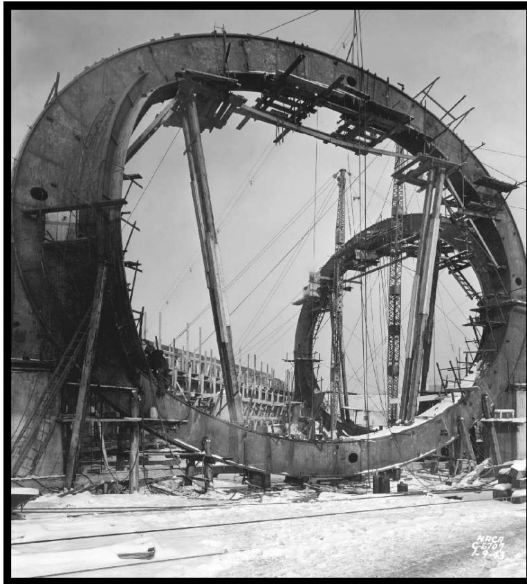
Figure 16.—Erection of the AWT corner ring in January 1943 (OH_Cuyahoga_Altitude-Wind-Tunnel_017).
