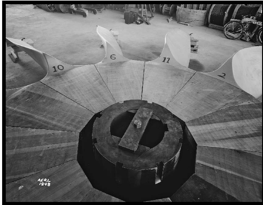
Figure 84.—Original 31'-0"-diameter spruce wood fan being assembled for the AWT in the Aircraft Engine Research Laboratory's hangar, 1943 (OH_Cuyahoga_Altitude-Wind-Tunnel_085).
