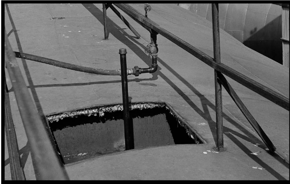
Figure 61.—Opening in the AWT's tunnel shell revealing a thin outer steel layer and fiberglass insulation, 1951 (OH_Cuyahoga_Altitude-Wind-Tunnel_062).
