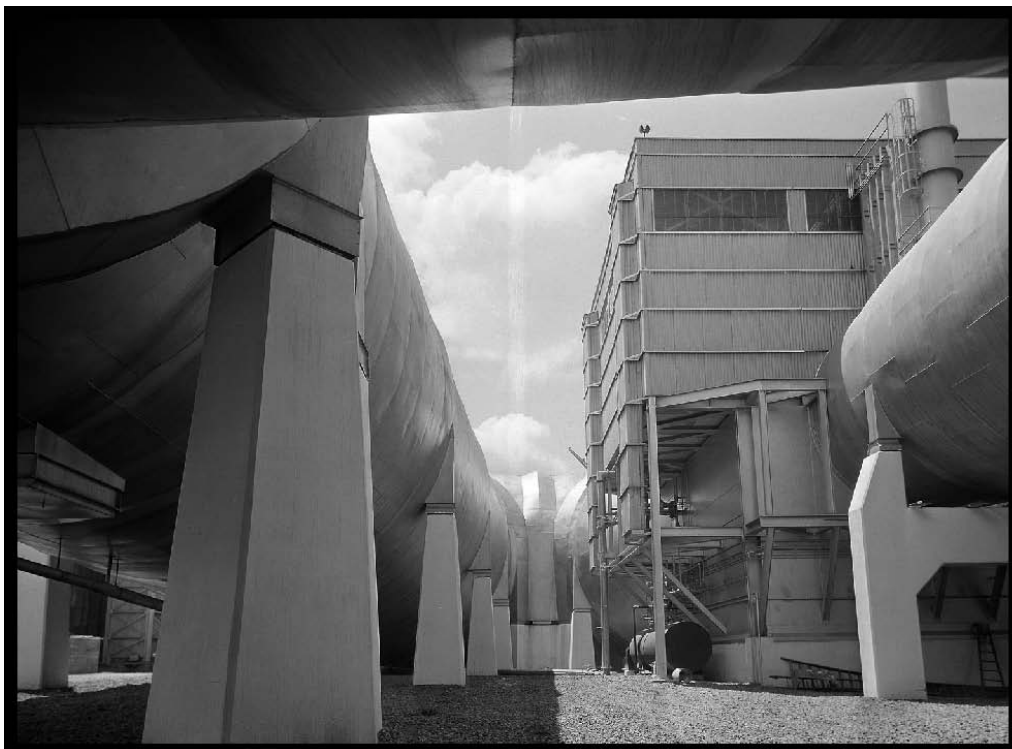
Figure 56.—Inside of the AWT loop showing the pylons and west-end concrete base (viewed from the east), 1945 (OH_Cuyahoga_Altitude-Wind-Tunnel_057).
