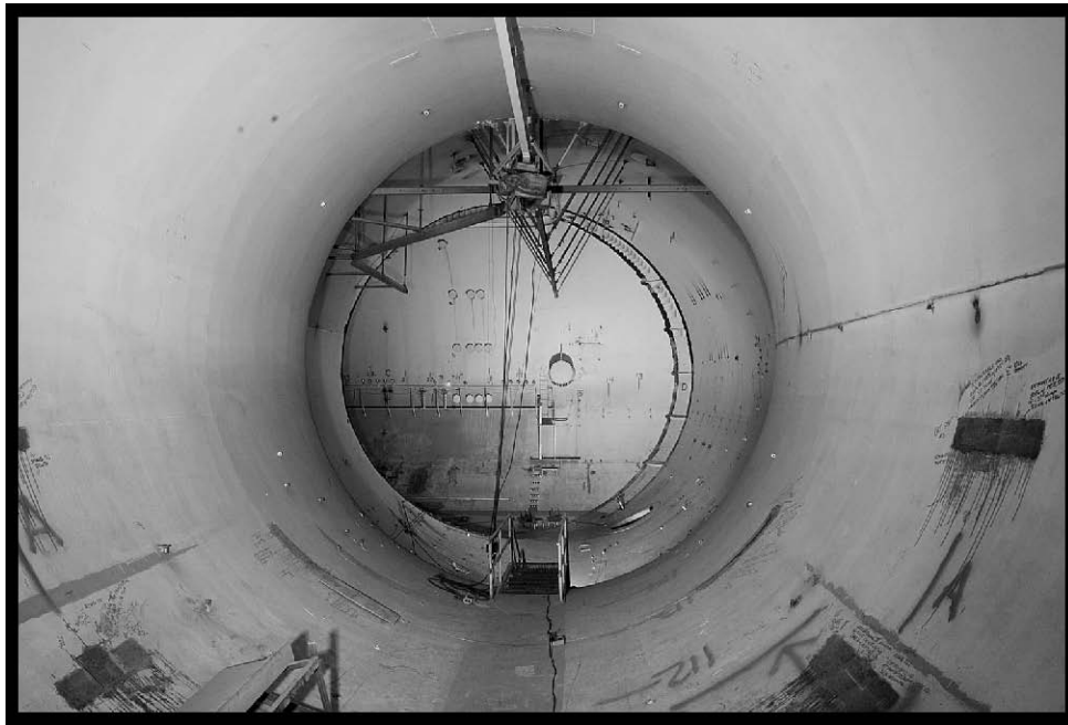
Figure 75.—Throat section in the northwest leg of the AWT (viewed from the east), 2007 (OH_Cuyahoga_Altitude-Wind-Tunnel_076).
