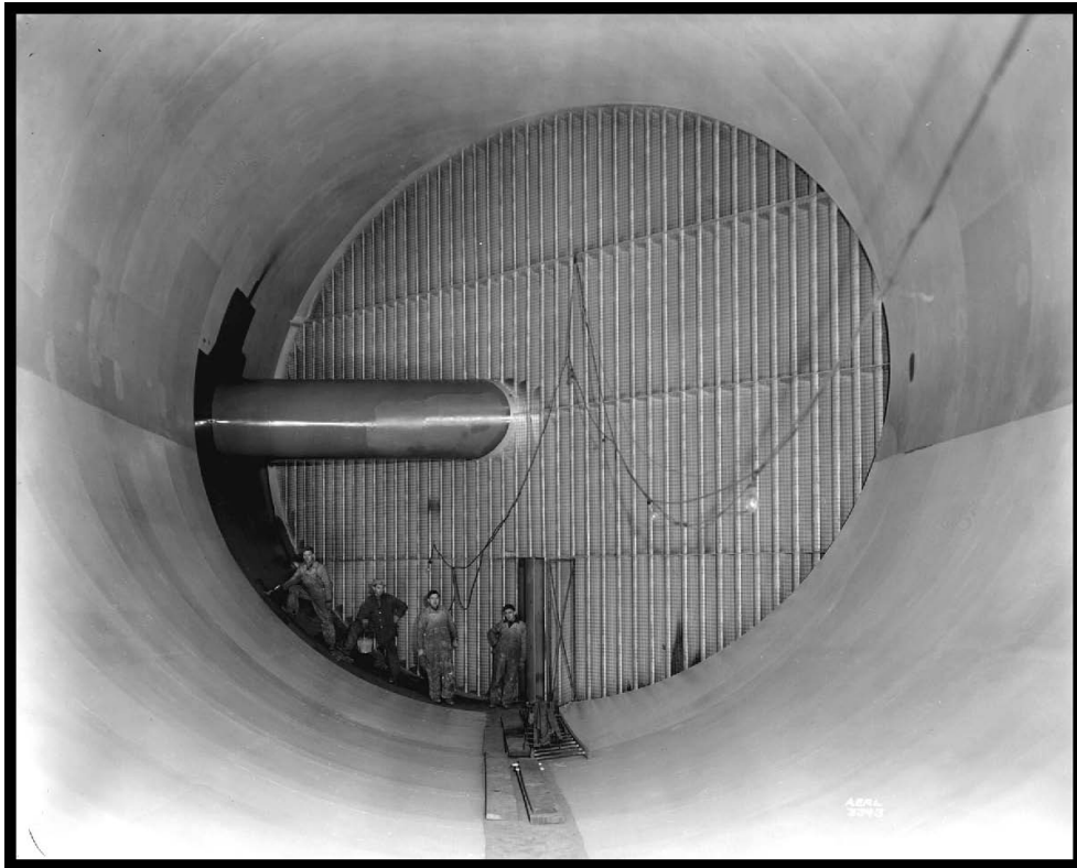
Figure 79.—Eastern leg of the AWT, showing a set of turning vanes and the fan's drive shaft (viewed from the north), 1944 (OH_Cuyahoga_Altitude-Wind-Tunnel_080).
