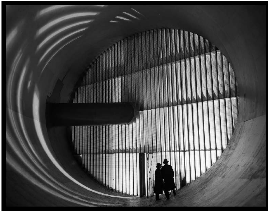
Figure 90.—Panel of turning vanes in the southeast corner of the AWT (viewed from the north), 1944 (OH_Cuyahoga_Altitude-Wind-Tunnel_091).
