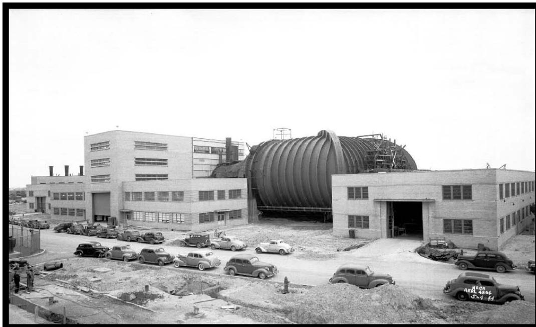
Figure 12.—Construction of the AWT as it neared completion, 1944 (OH_Cuyahoga_Altitude-Wind-Tunnel_013).
