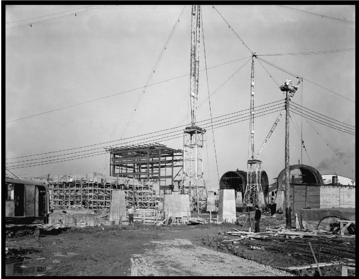
Figure 15.—Pylons for the AWT, along with steel framing for the Shop and Office Building (viewed from the southwest), 1942 (OH_Cuyahoga_Altitude-Wind-Tunnel_016).
