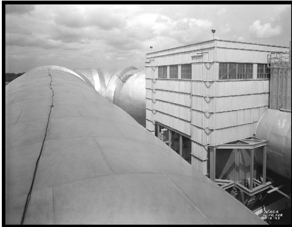
Figure 44.—AWT and test chamber before walkways were installed (viewed from the southeast corner), 1945 (OH_Cuyahoga_Altitude-Wind-Tunnel_045).
