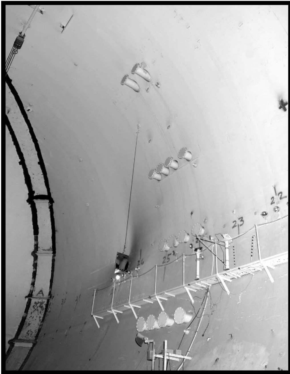
Figure 72.—Western wall of the AWT showing sealed penetrations for the refrigeration lines to the cooling coils, 2005 (OH_Cuyahoga_Altitude-Wind-Tunnel_073).
