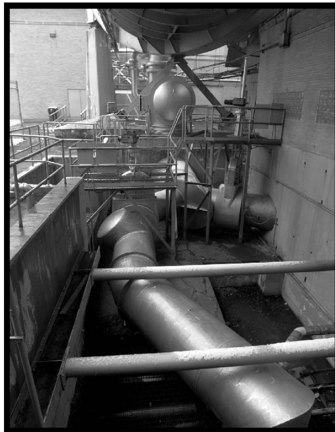
Figure 97.—Cooler pit under the northeast section of the tunnel (viewed from the west), 2007 (OH_Cuyahoga_Altitude-Wind-Tunnel_098).
