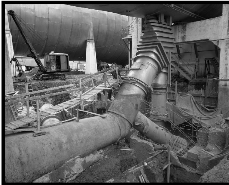
Figure 96.—Original exhaust scoop underneath the northeast section of the tunnel, 1951 (OH_Cuyahoga_Altitude-Wind-Tunnel_097).
