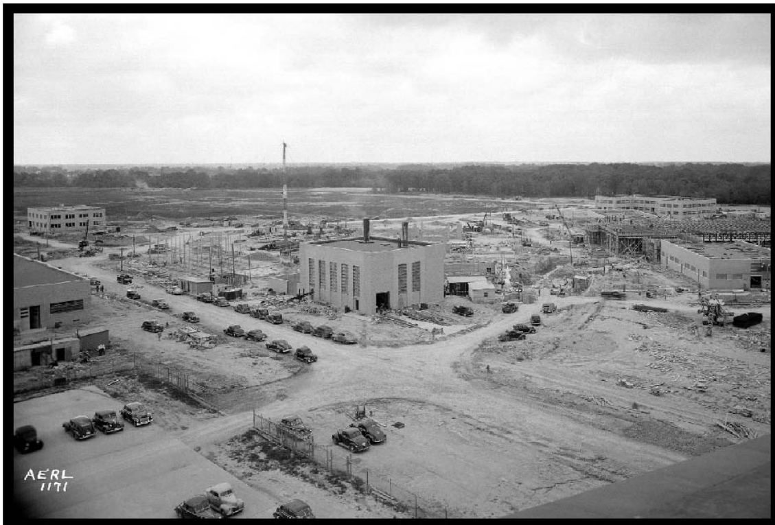
Figure 14.—Construction of the AERL near the site of the AWT, 1942 (OH_Cuyahoga_Altitude-Wind-Tunnel_015).
