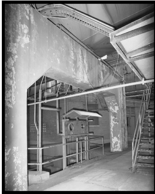
Figure 59.—H-shaped concrete support under the tunnel as it exits the east wall of the test chamber, 2005 (OH_Cuyahoga_Altitude-Wind-Tunnel_060).
