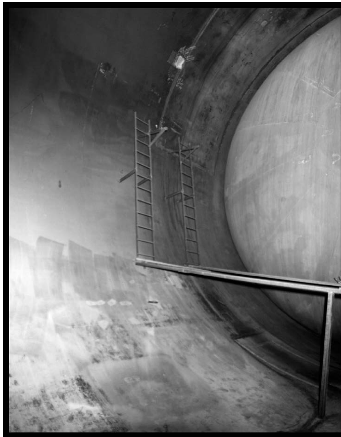
Figure 68.—Interior of the AWT south leg where the drive fan was formerly located, 2005 (OH_Cuyahoga_Altitude-Wind-Tunnel_069).
