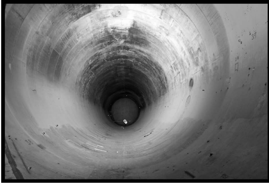
Figure 67.—South leg of the AWT (viewed from the west), 2007 (OH_Cuyahoga_Altitude-Wind-Tunnel_068).
