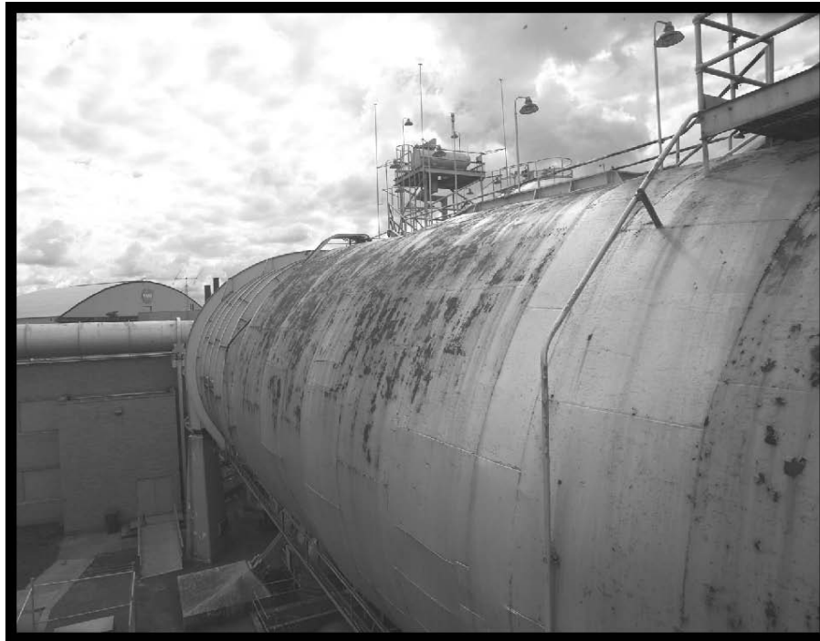
Figure 50.—Northeast leg of the AWT (viewed from the west), 2005 (OH_Cuyahoga_Altitude-Wind-Tunnel_051).
