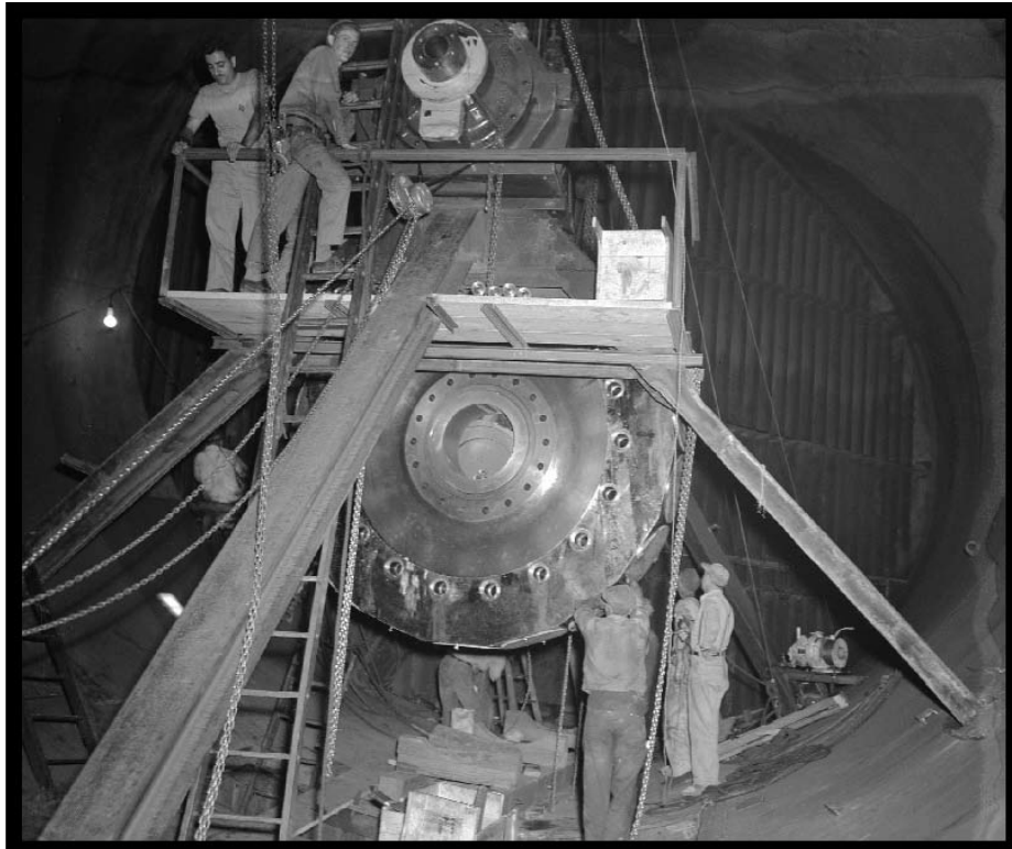
Figure 86.—New fan hub being installed near the southeast corner of the AWT, 1951 (OH_Cuyahoga_Altitude-Wind-Tunnel_087).
