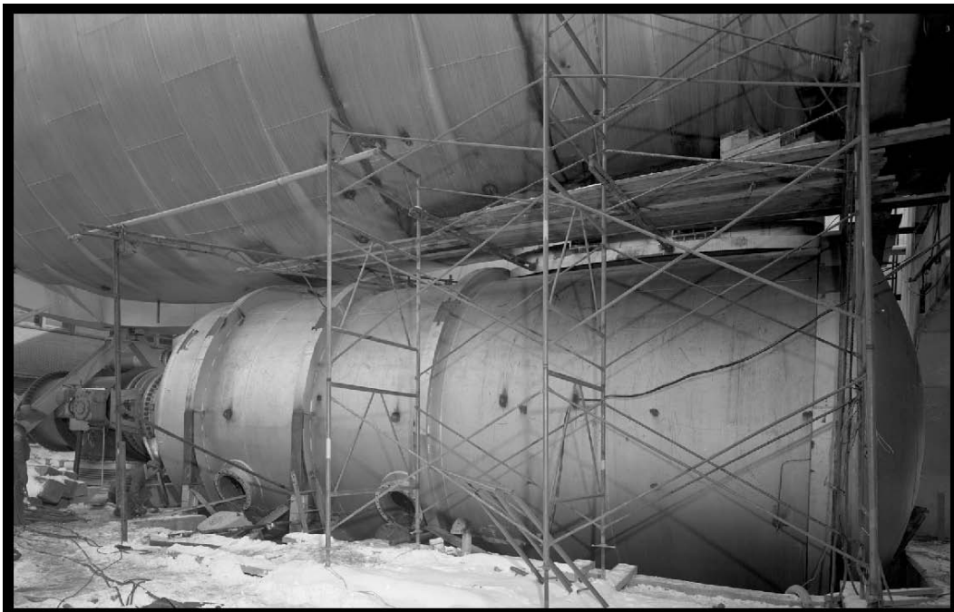
Figure 23.—Installation of a new exhaust gas cooler underneath the northeast section of the AWT, 1951 (OH_Cuyahoga_Altitude-Wind-Tunnel_024).
