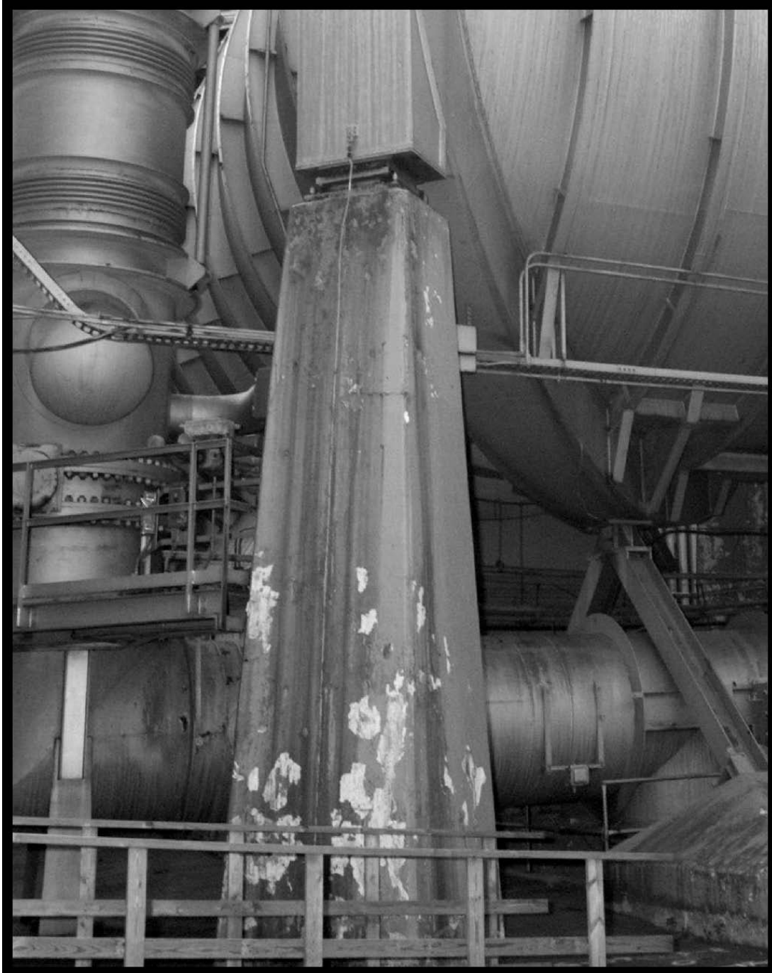
Figure 54.—Concrete pylon supporting the northeast corner of the AWT, with rollers exposed between the concrete and steel, 2005 (OH_Cuyahoga_Altitude-Wind-Tunnel_055).
