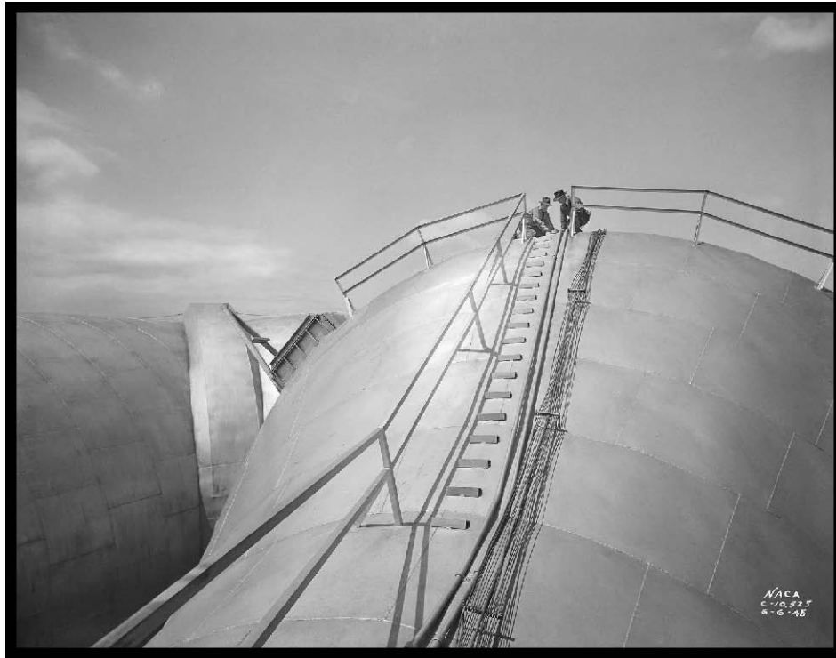
Figure 46.—Throat section of the northwest corner of the AWT (viewed from the east), 1945 (OH_Cuyahoga_Altitude-Wind-Tunnel_047).
