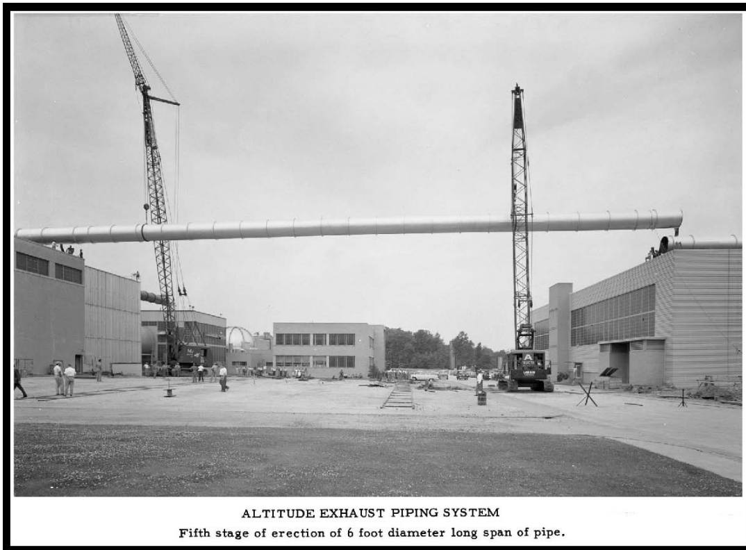
Figure 24.—Erection of pipe connecting NACA Lewis' new test facilities to the AWT's and Engine Research Building's exhausters, 1957 (OH_Cuyahoga_Altitude-Wind-Tunnel_025).
