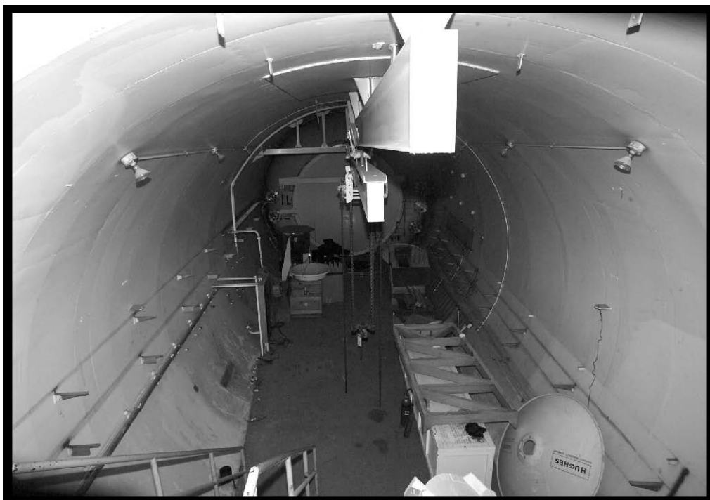
Figure 78.—Test section after the air scoop was removed (viewed from the west through the northeast tunnel section), 2005 (OH_Cuyahoga_Altitude-Wind-Tunnel_079).
