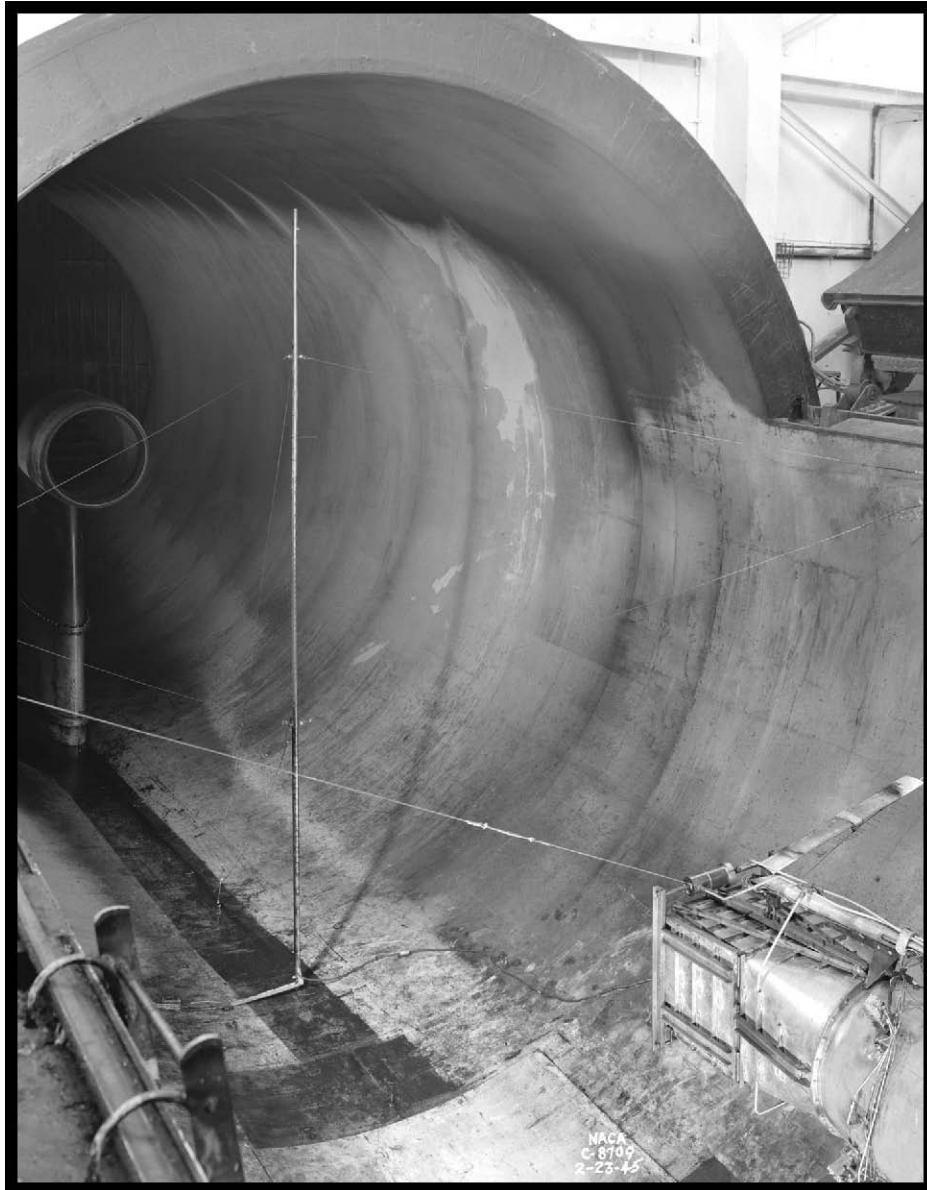
Figure 95.—View from the test section showing the exhaust scoop downstream, 1945 (OH_Cuyahoga_Altitude-Wind-Tunnel_096).
