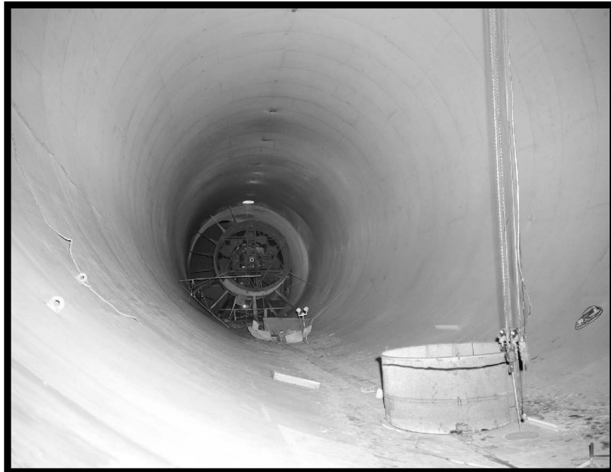
Figure 65.—Interior of the south leg of the AWT, with the fan without its fairing at the far end (viewed from the east), 1961 (OH_Cuyahoga_Altitude-Wind-Tunnel_066).
