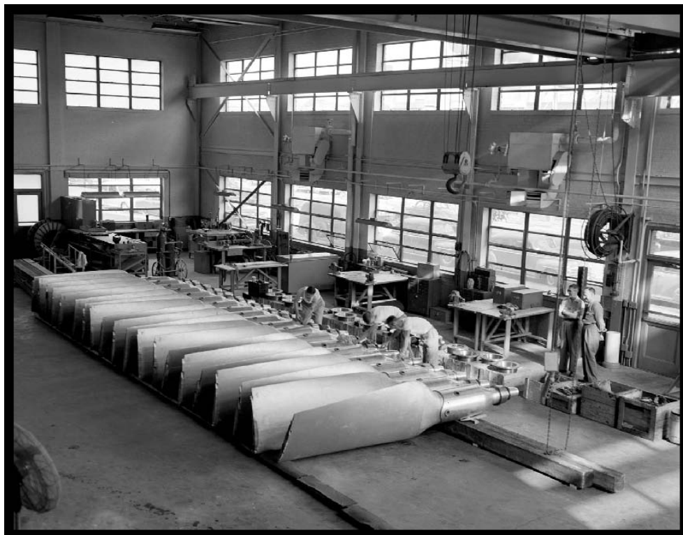
Figure 85.—New blades being prepared in the AWT shop area for installation in the tunnel, 1951 (OH_Cuyahoga_Altitude-Wind-Tunnel_086).
