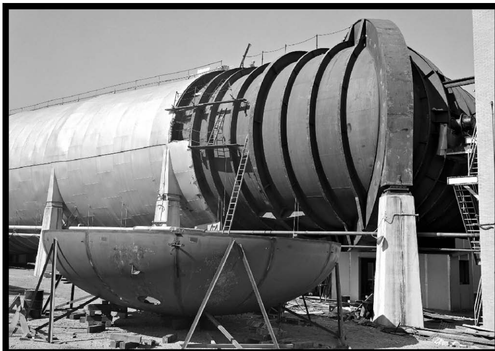
Figure 60.—Southeast corner of the AWT showing a thin outer shell (left) and a thicker inner shell and support rings (right), 1961 (OH_Cuyahoga_Altitude-Wind-Tunnel_061).
