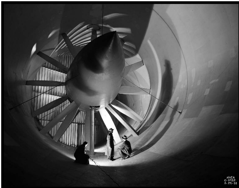
Figure 82.—Original AWT fan, tail fairing, and supports, showing a set of turning vanes behind (viewed from the west), 1944 (OH_Cuyahoga_Altitude-Wind-Tunnel_083).
