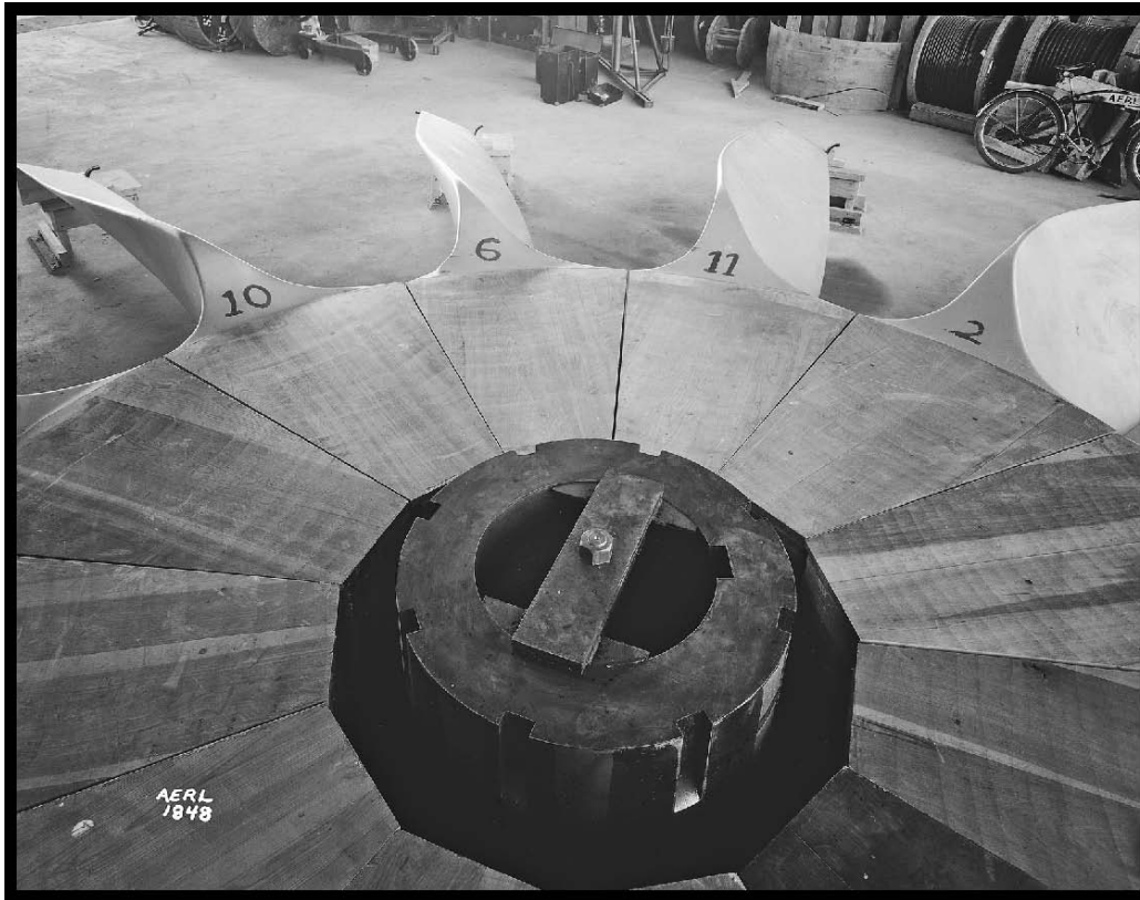
Figure 20.—Assembly of the 32'-0"-diameter spruce wood fan in the Aircraft Engine Research Laboratory's hangar prior to the fan's installation in the AWT, 1943 (OH_Cuyahoga_Altitude-Wind-Tunnel_021).
