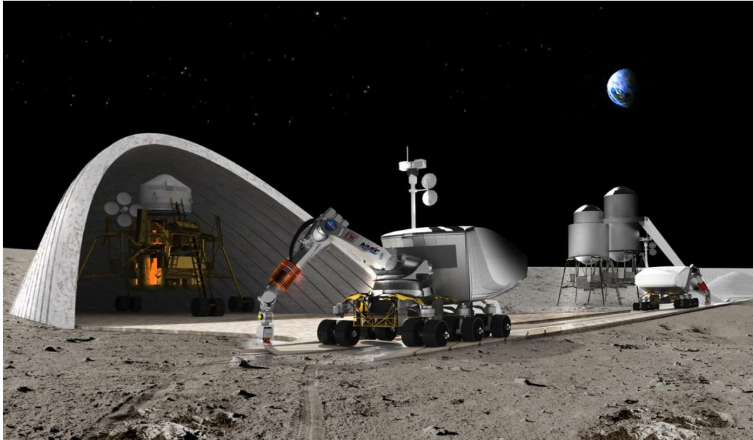
Figure 2. A Contour Crafting robot is shown here printing a road in front of a parabolic hangar structure housing a lunar lander. In the background can be seen a plant intended for processing regolith that will be used in the construction process.
