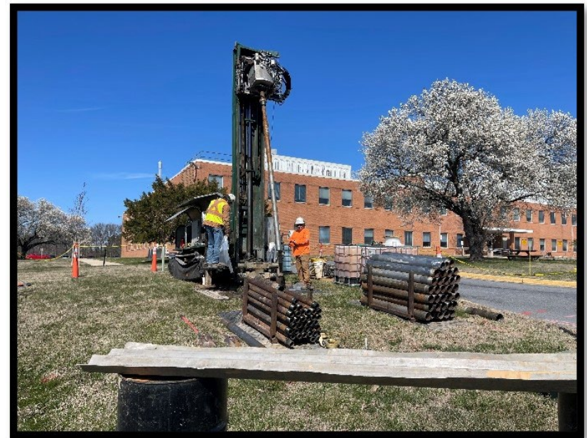
Drilling during Site Investigation
