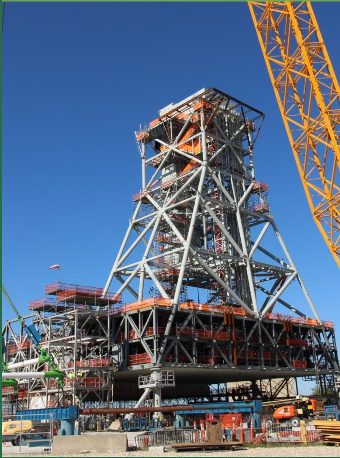
Mobile Launcher 2 Rig & Set 1.5 Weeks Ahead of Schedule; Tower Mod 4 Installed
