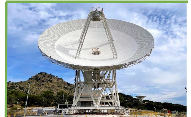
Deep Space Station 53 is a new waveguide antenna that went online in February 2022 at NASA's Deep Space Network's ground station in Madrid
