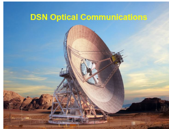
Figure 11.34: Artist overlay of built DSN RF antenna and planned 8m optical segments at its center. Credit: NASA.
