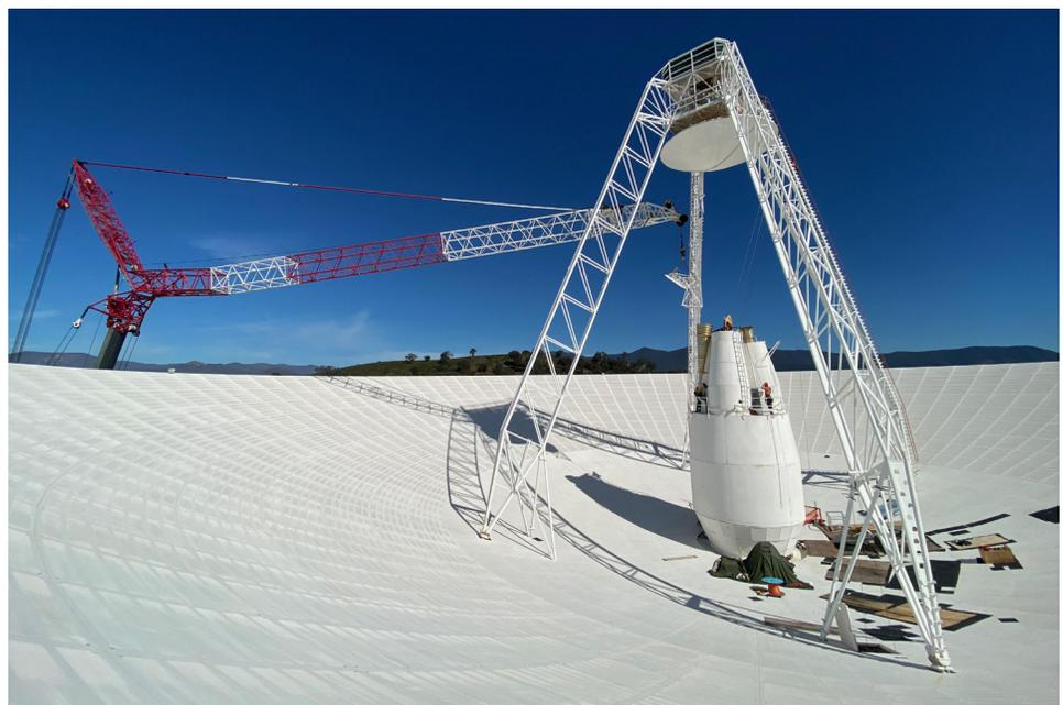
*Inside a 70-meter antenna at the DSN Deep Space Station in Canberra, Australia. NASA/JPL-Caltech*
