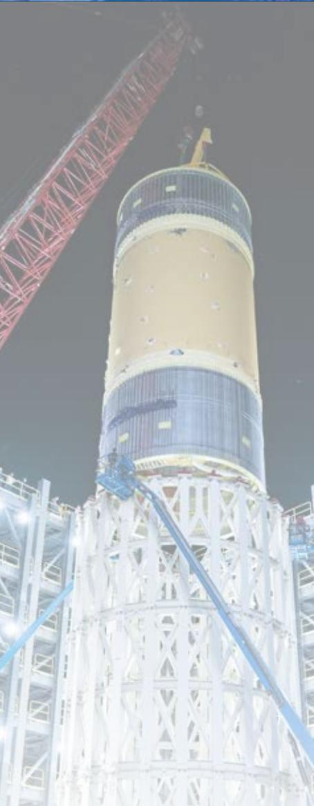
*NASA's Space Launch System (SLS) core stage is installed in Test Stand 4697 at NASA's Marshall Space Flight Center in Huntsville, Alabama in July 2019. (NASA/Boeing)*
