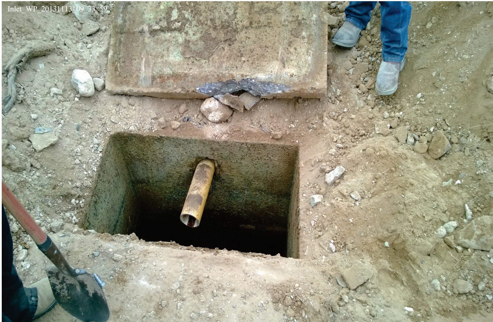
Photograph showing the inlet pipe (from Building 114 to the septic tank) for SWMU 22.
