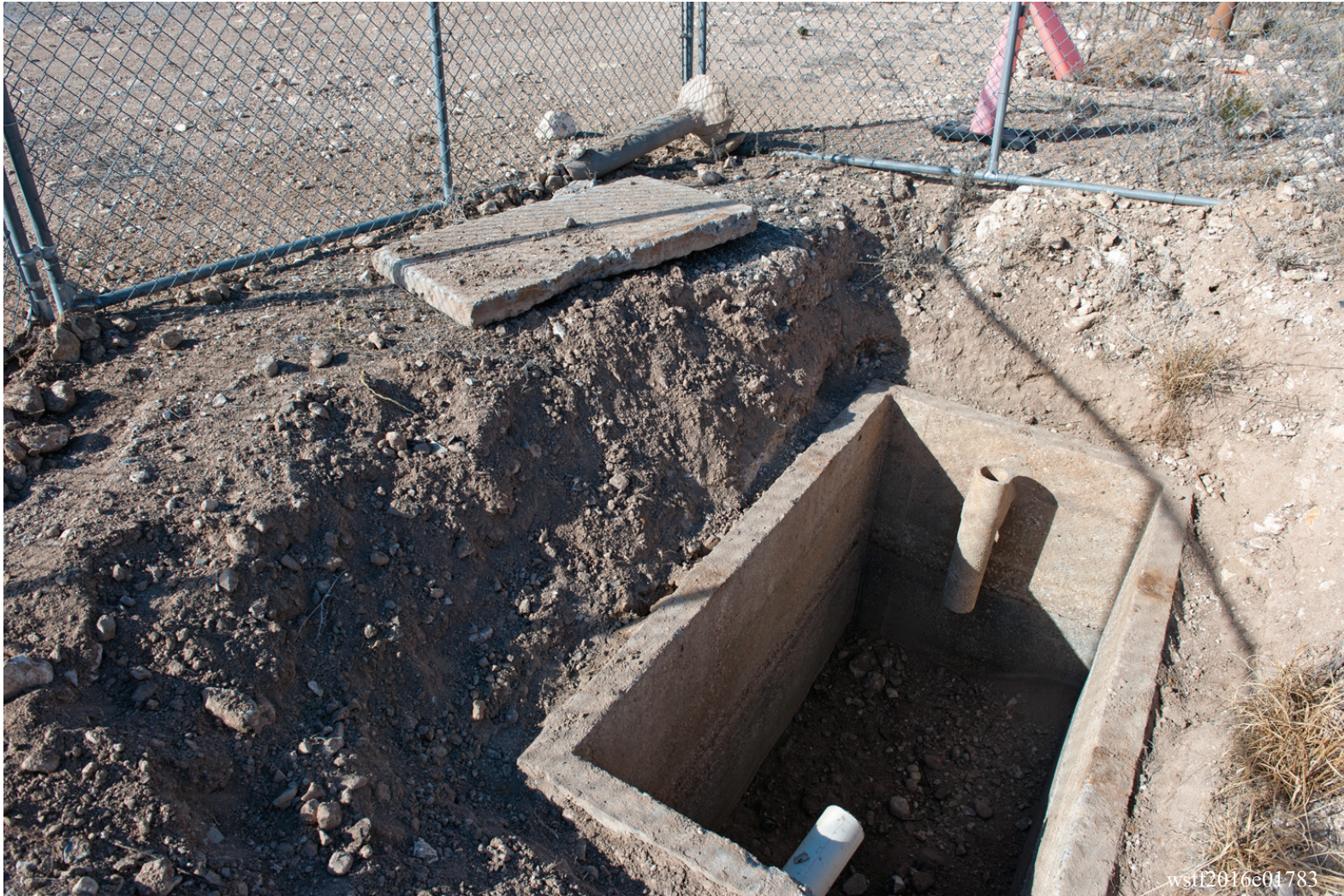
Building 114 (SWMU 22) septic tank. The surface vent can be seen with the tank top at the upper left of the photo. This photo was taken prior to removal of the tank. The tank contained no bottom.
