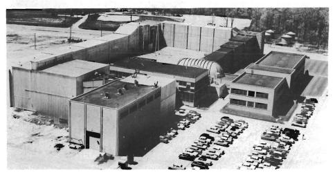
The erection of a duct which permits reuse of air within the tunnel is the left hand portion of the 8x6 tunnel pictured here. The test section is inside the dome near the center of the photo.
