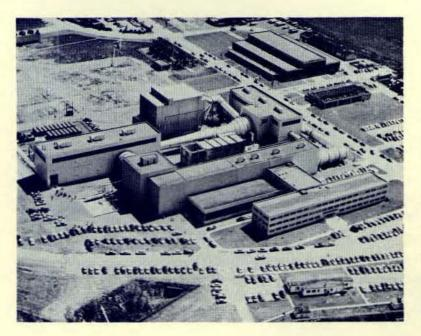
The steel air duct at right leads to the tunnel test section, housed in the long, narrow structure in the center. The building at left and the one at the opposite end of the intervening steel duct house axial flow compressors, which supply the air flow. Seven electric motors totaling 250,000 HP, drive the compressors. Flanking the center ducting are an air dryer (top center) and an acoustic muffler (center). Offices and shops are housed in the building area in the lower part of the photograph.
