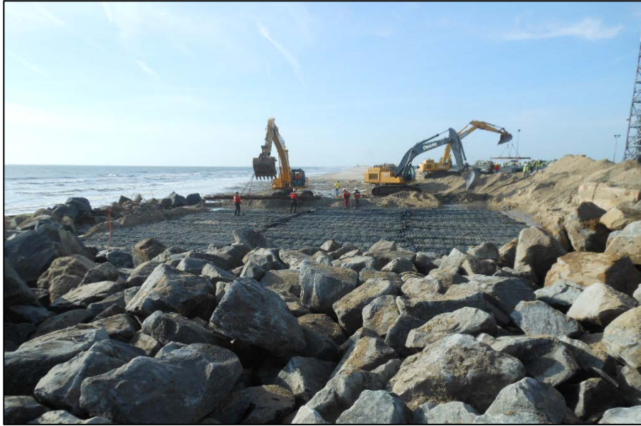
Figure 2-3: Installation of Marine Mattresses
