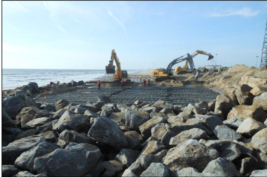
Figure 2-3: Installation of Marine Mattresses
