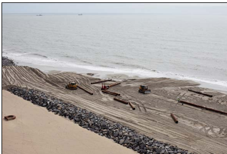
Figure 2-7: Bulldozers Grading Newly Discharged Sand
