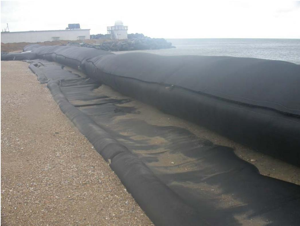
Figure 3-9. Scour apron exposed on landward side of Geotube™ at northern end of structure.
