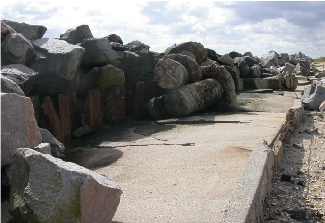
Figure 3-15. Remnants of concrete apron with steel sheet pile wall.
