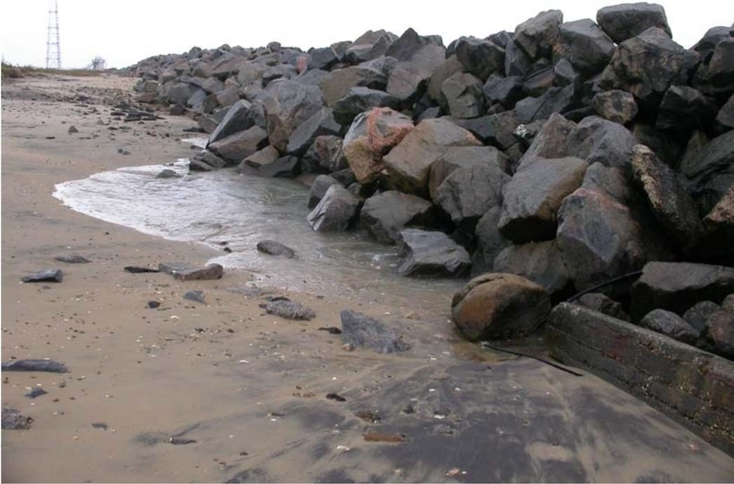
Figure 3-16. Water flowing through seawall by wave action.
