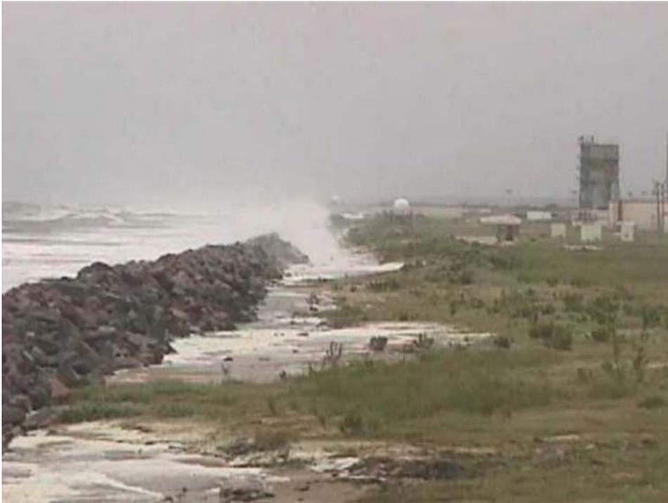
Figure 2-15. Rock seawall during Hurricane Dennis, September 1999.
