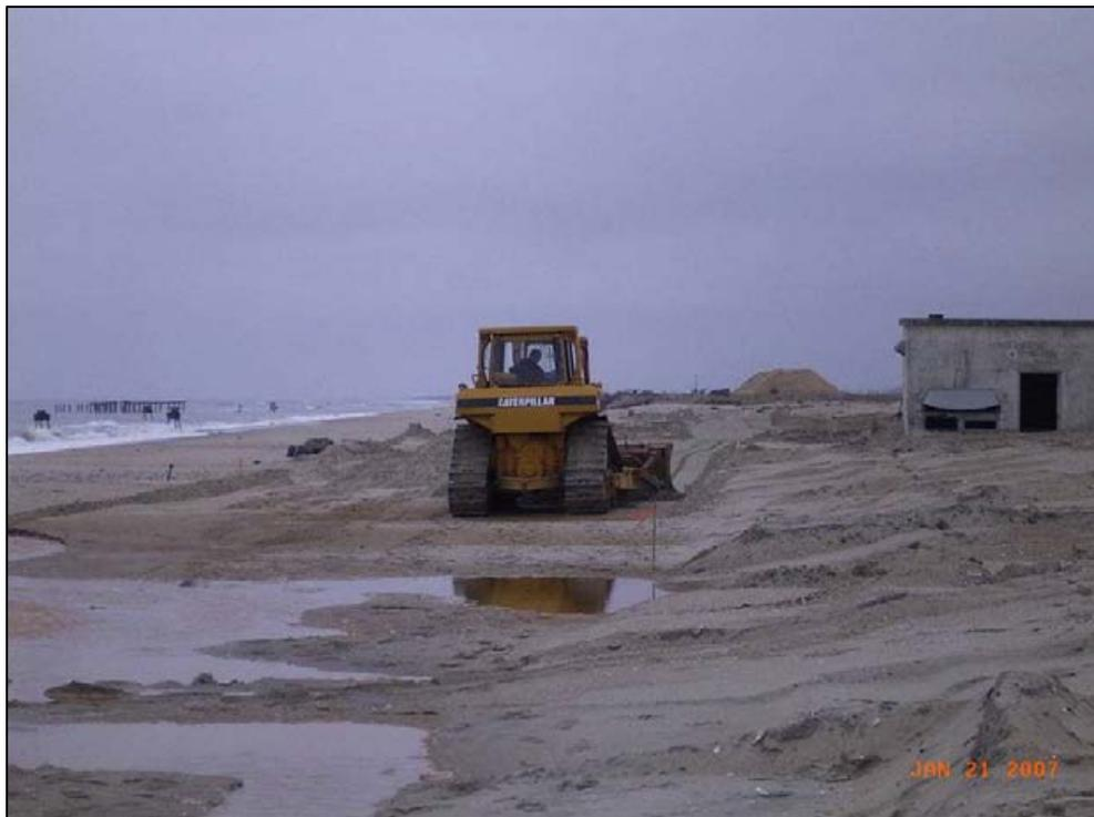
Plate 6-4. Geotextile Tube Corridor Grading, Facing South
