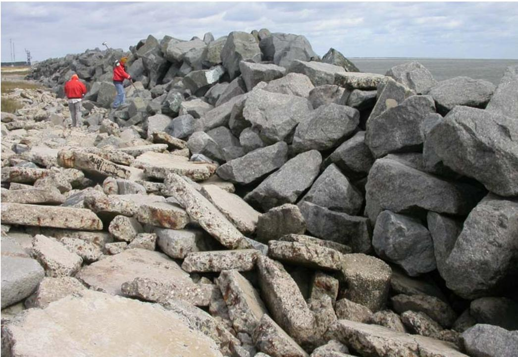
Figure 3-17. Rubble pile behind seawall, presumably to fill scour hole.
