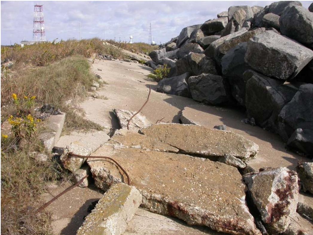
**Figure 3-13. Washout under the concrete apron causing cracking and tilting.**
