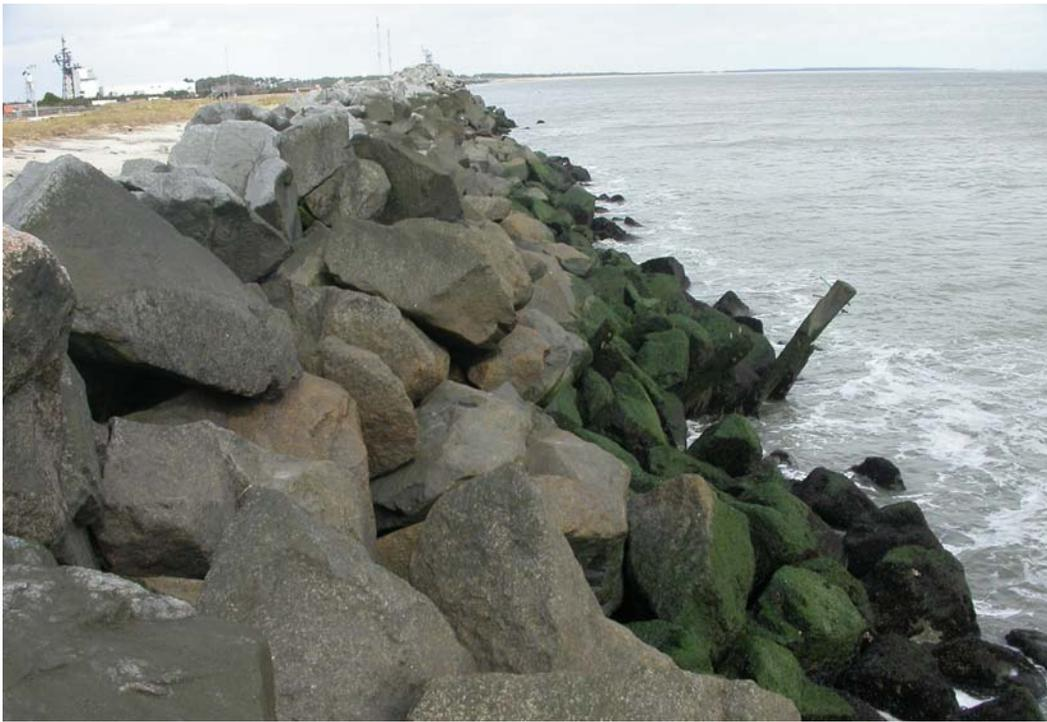
Figure 3-12. Steep seaside face on seawall.
