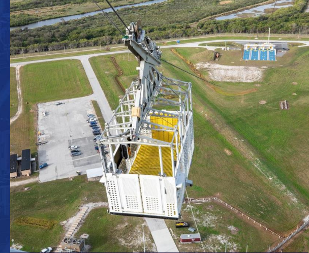
EGS teams begin installation of four emergency egress baskets at Launch Complex 39B.
