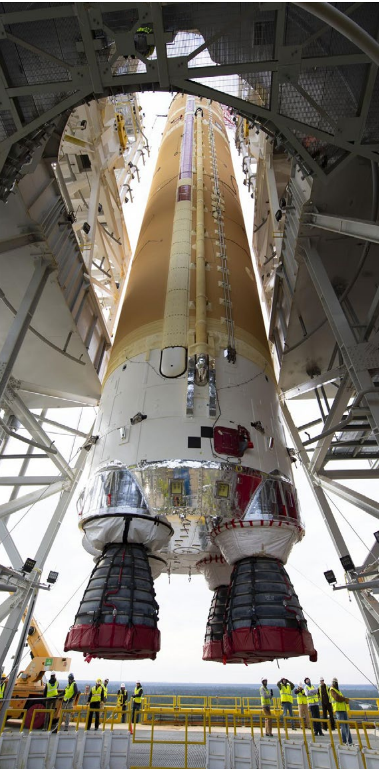
Installing SLS rocket onto the B-2 Test Stand.
