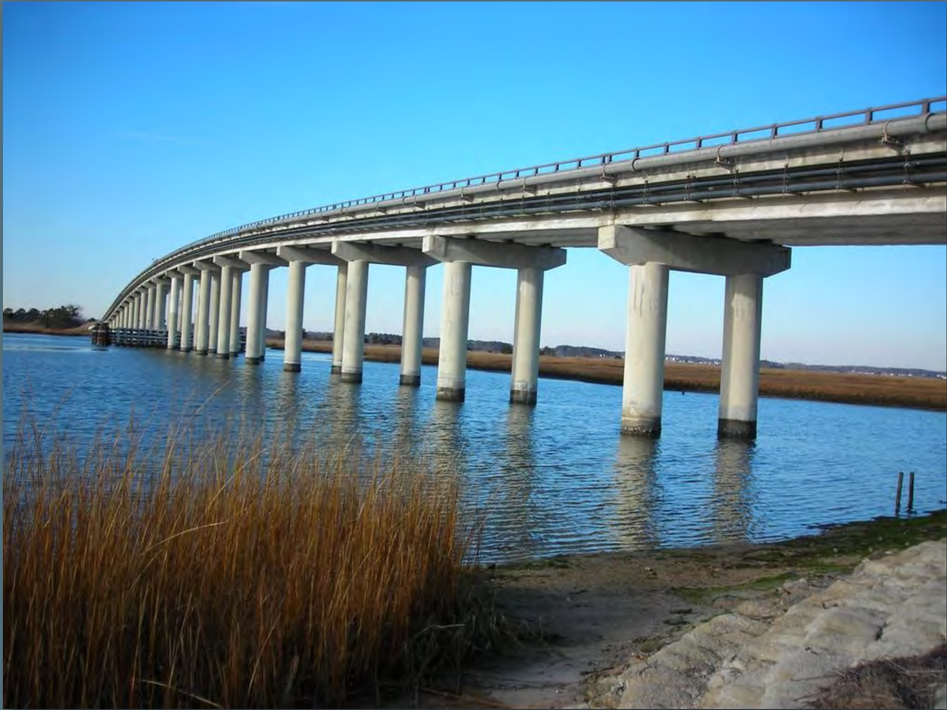
Causeway Bridge The 1960’s era bridge is at the end of its design life. A new causeway bridge would be constructed parallel to the existing structure prior to its removal.
