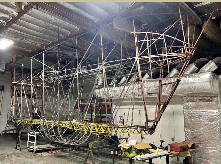
Completed new build gondola frames mated with frames salvaged from 1943 crash; note beginning of keel framing
