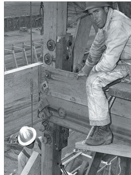
Hangar Two under construction
