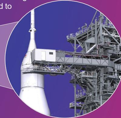
The **crew access arm** and **Orion service module umbilical** are located 40 feet higher on mobile launcher 2.
