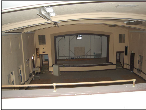
Figure 4-3. Interior of Building 25's auditorium before renovation.
