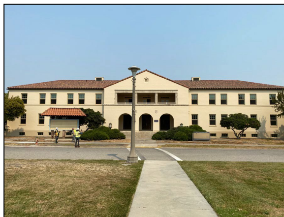
Figure 4-7. Exterior of Building 25 at ARC after renovation.
