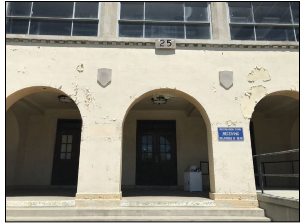
Figure 4-5. Exterior entry of Building 25 at ARC prior to renovation.
