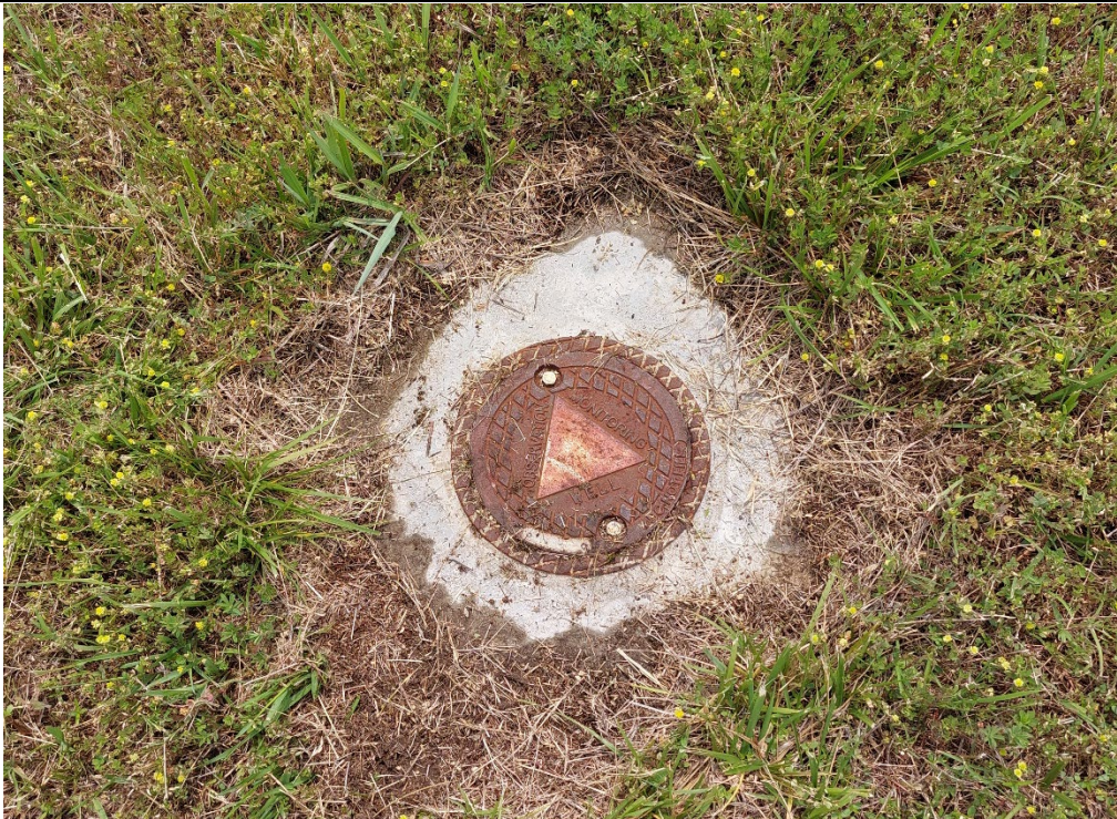
View of FFTA-MW109. Flush mount completion in grass on south side of abandoned taxiway.
