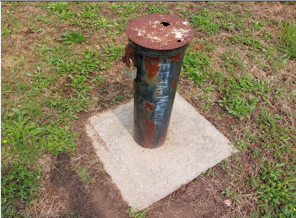
View of FFTA-MW101S. The protective casing's cap has rusted through and needs replaced.
