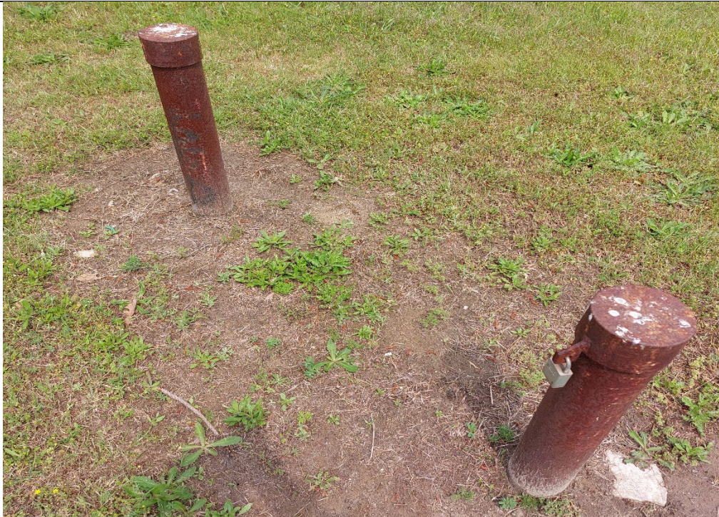
View of FFTA-MW055S and FFTA-MW055D. Other than some rust the well are in good condition.
