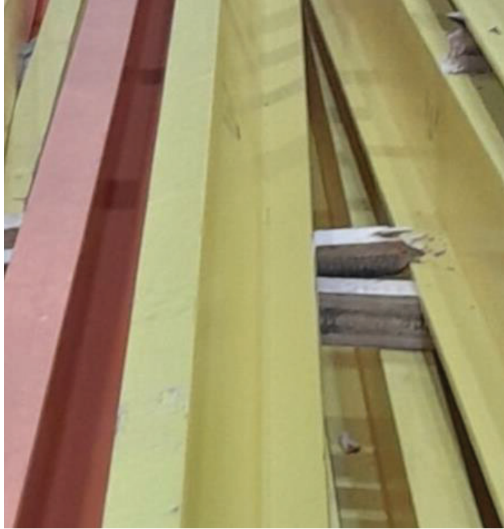
Figure 8: View of broken dunnage under beam.
