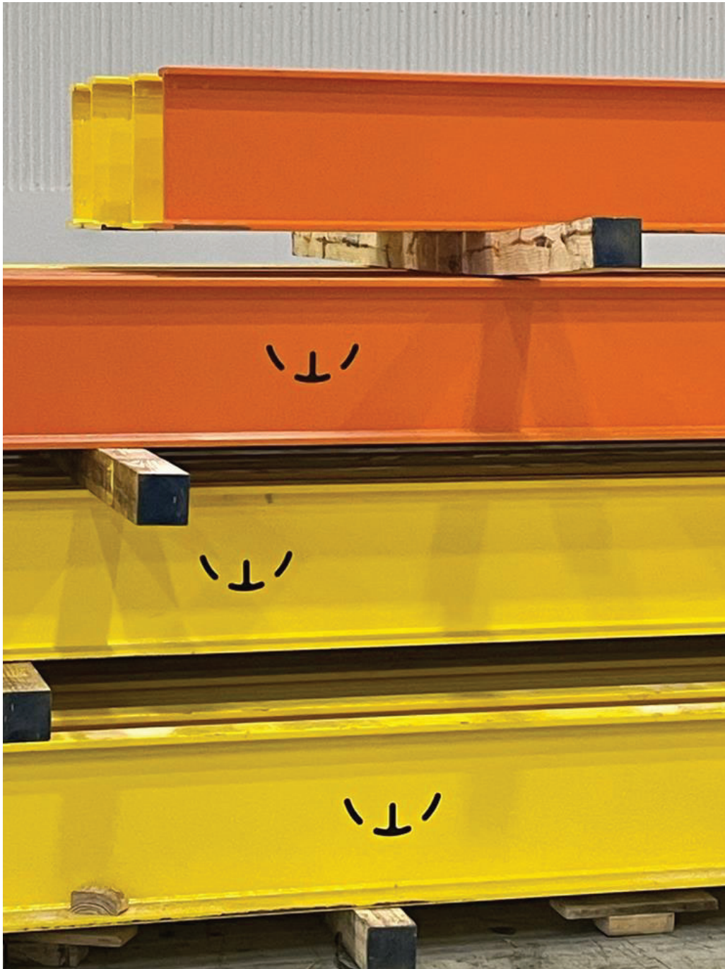
Figure 24: Misaligned dunnage supporting steel beams.
