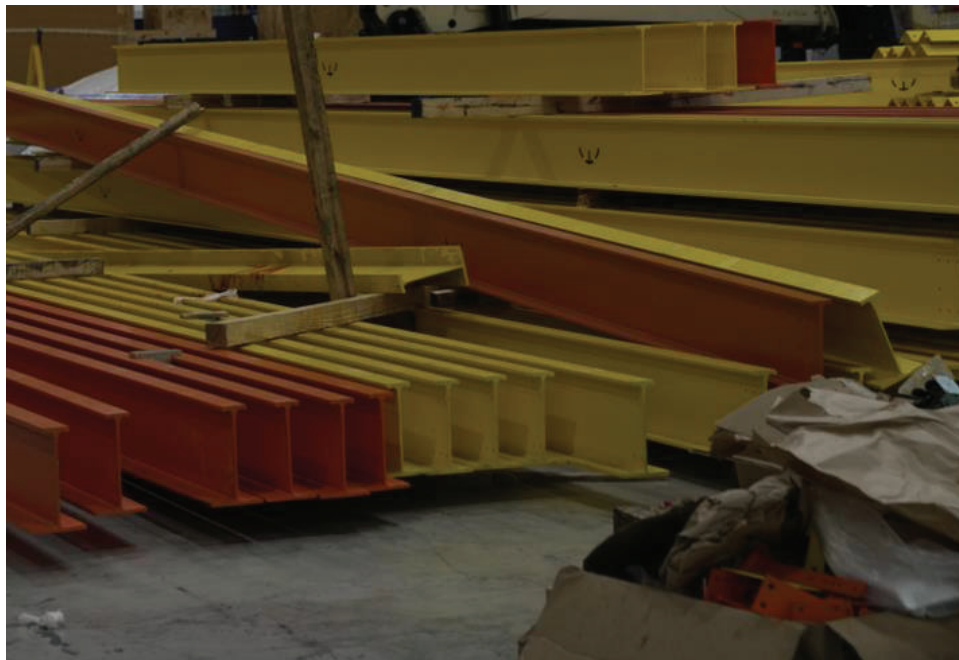
Figure 9: View of collapsed beams.
