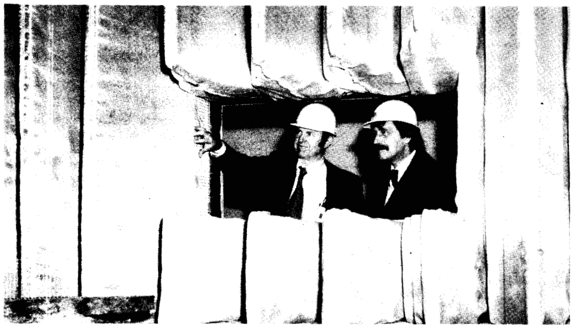
Neel D. Fauber (left) and Erwin M. Lauffer examine acoustic baffle wall construction in the new Engine Fan and Jet Noise Facility.
