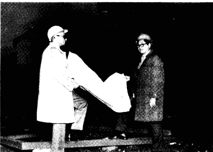
Paul Weisenbach (left) and Suey T. Yee go over construction plans for rehabilitating the Equipment Utilization Building.
