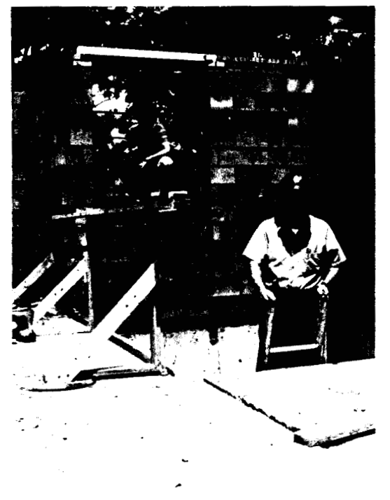
Bill Schoren (foreground) and Roger Rachul, Construction Engineering, determine Control Building progress.
