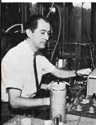
Dr. William L. Fielder resets instrumentation in studies of the electrical conductivity of a variety of ionic compounds to reveal the mechanism of ion transport in the solid state.
